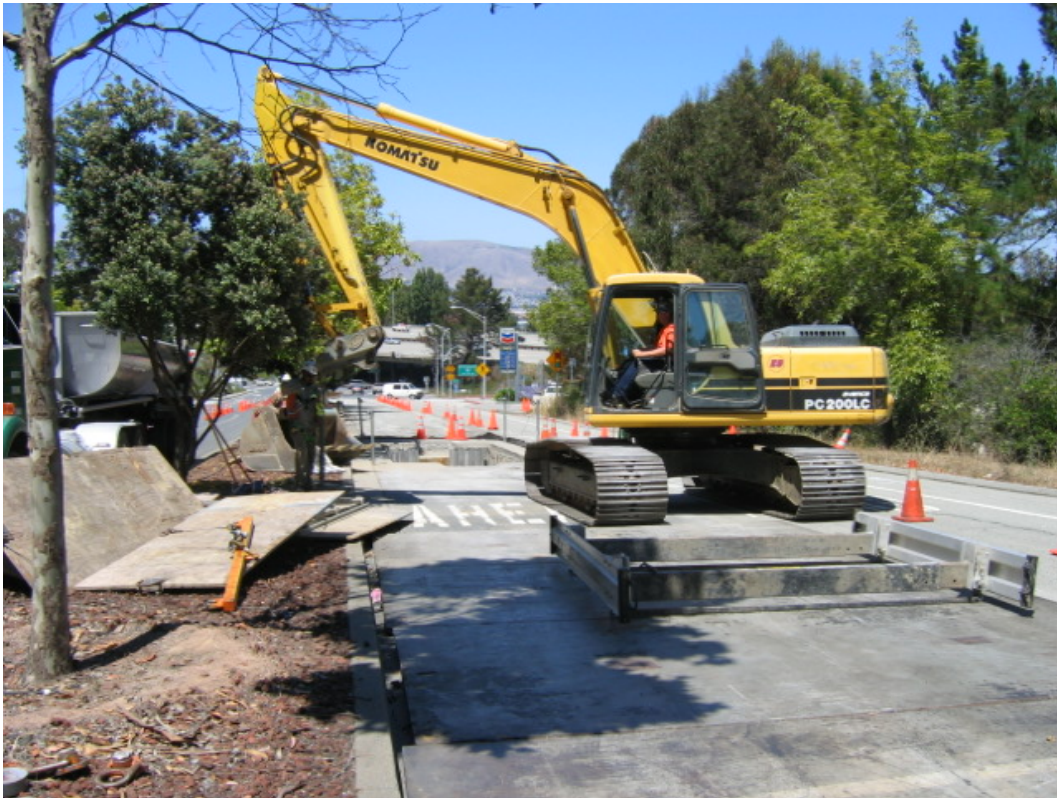
Figure 3 – Excavation of Manhole #42 along San Bruno Ave, Segment 3, July 20, 2005.
