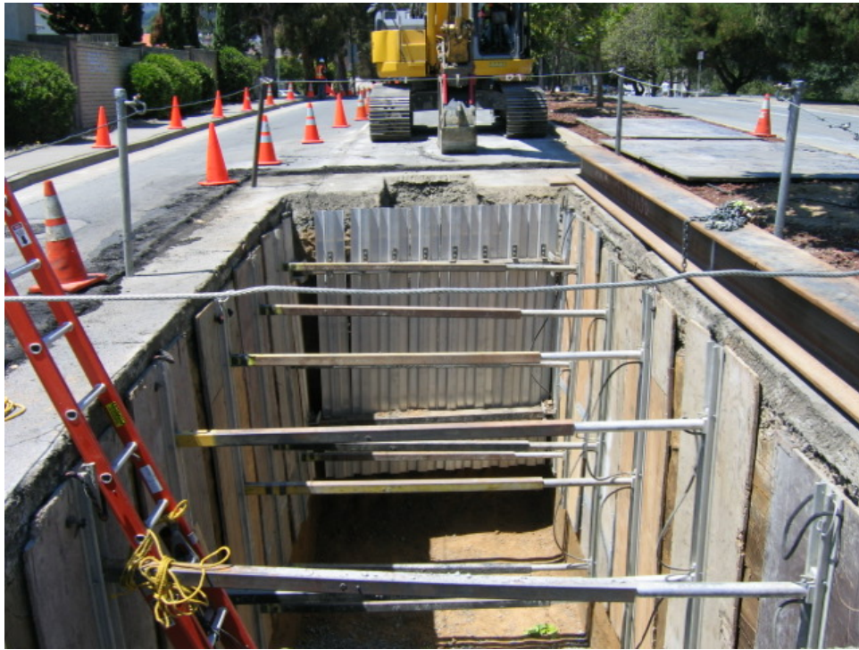
Figure 3 – Excavation of Manhole #43 along San Bruno Ave, Segment 3, July 27, 2005.
