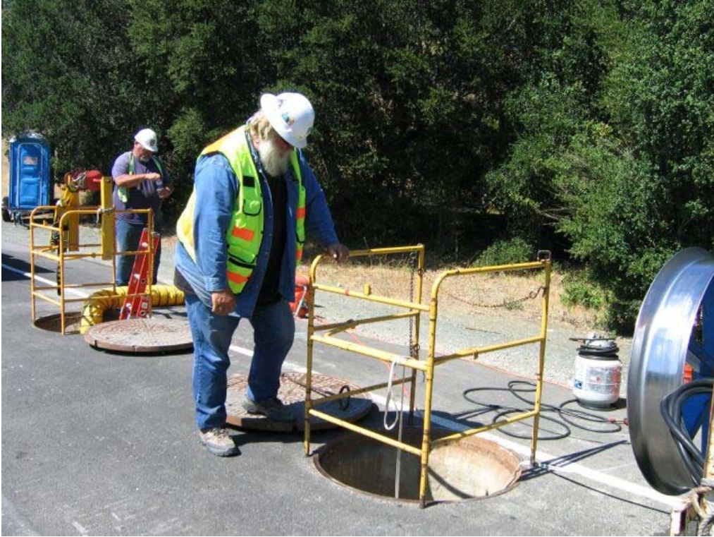
Figure 1 – Crews conducting jacket testing on installed cable, Segment 1, July 28, 2005
