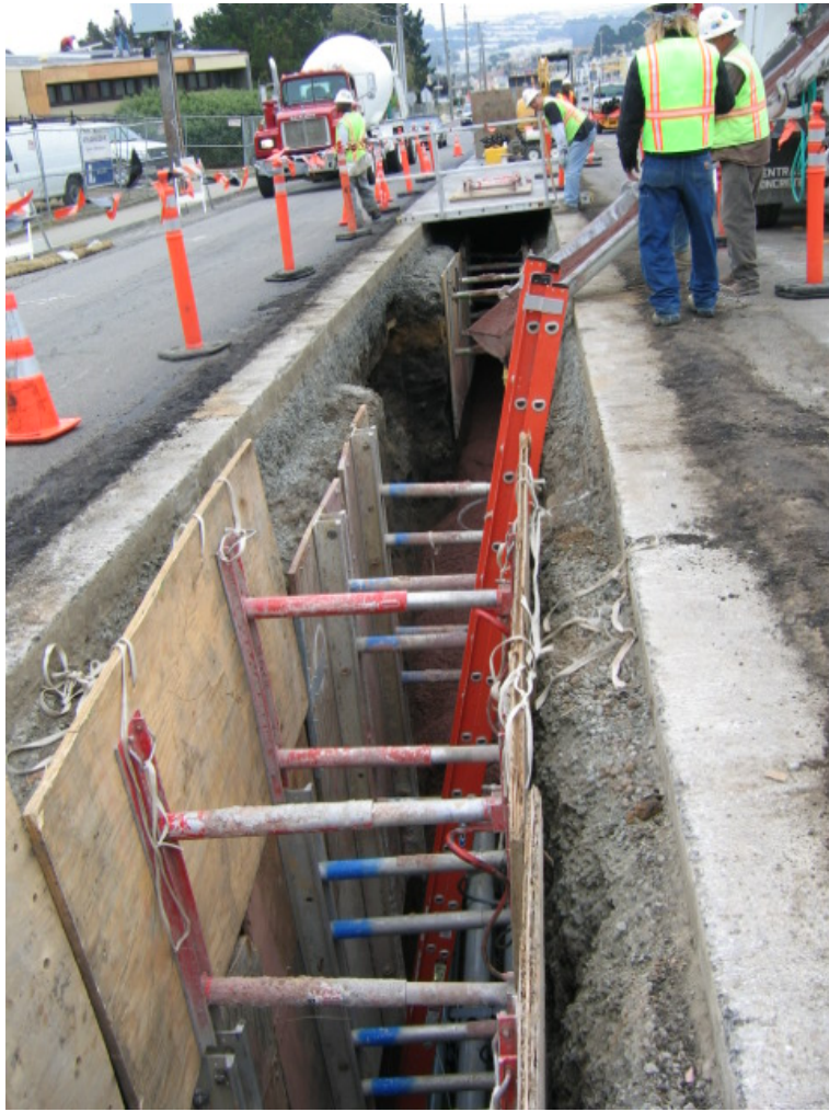
Figure 5 – Trenching operations on East Market in Daly City, Segment 5, July 27, 2005.
