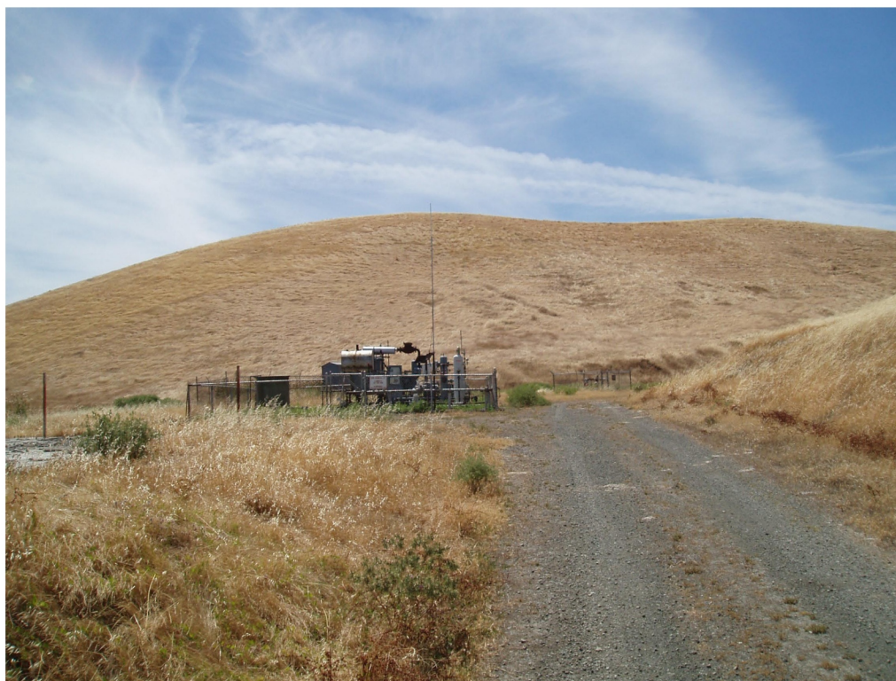
Kirby Hills Well Site S-2 and Temporary Compressor Location
