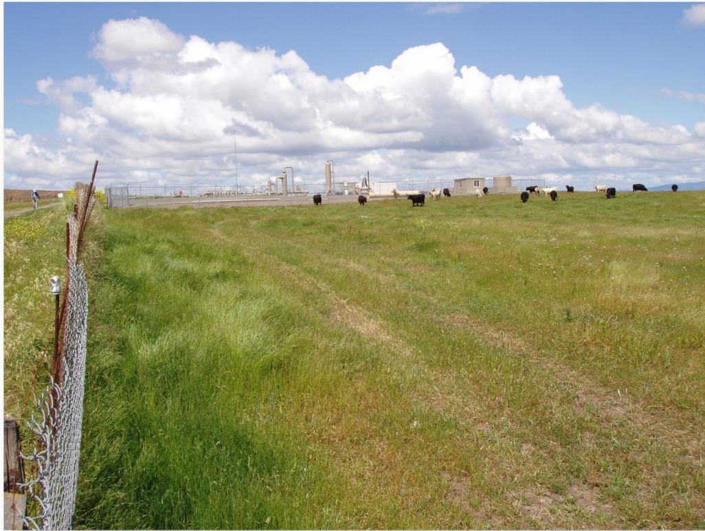
Calpine's Existing Metering and Dehydration Station (Photo is Looking West From Existing Access Road)
