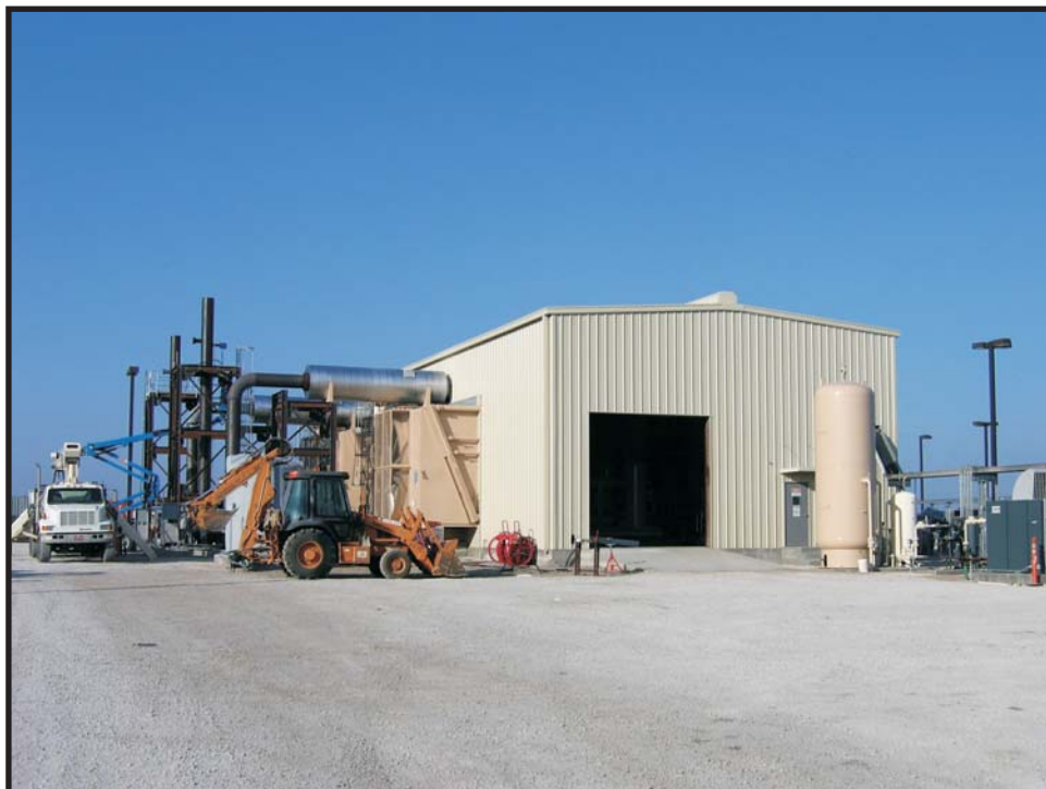
Compressor Building at the existing Kirby Hills Compressor Station Facility, January 23, 2007
