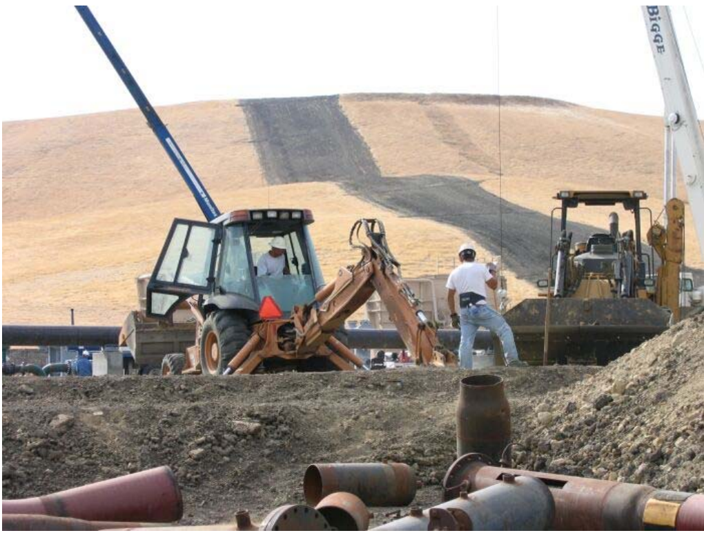
Figure 4 – Crews working at Compressor Station, September 26, 2006.
