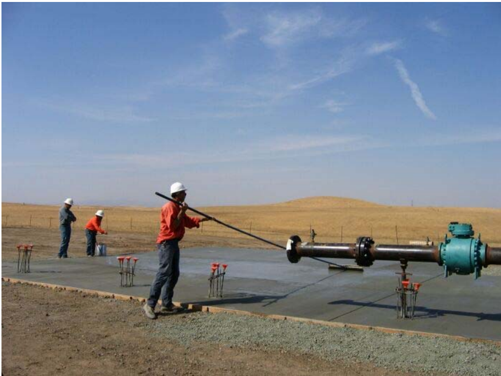
Figure 5 – PG&E working on building foundation at the Metering Station, September 28, 2006.
