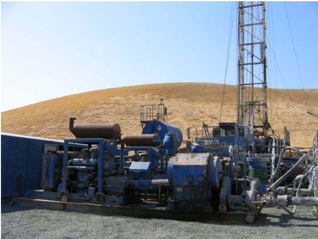
Figure 2 – East side of drill rig at well site S-2, September 26, 2006.
