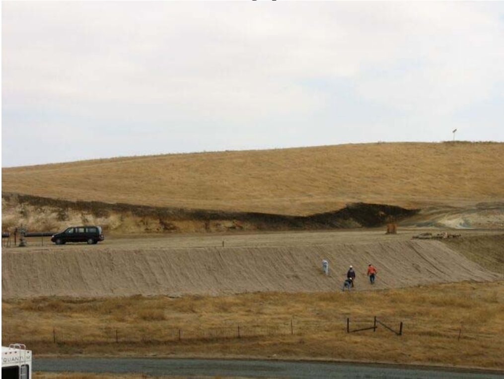
Figure 1 – Erosion controls (jute matting) being installed at well site S-1, October 5, 2006.
