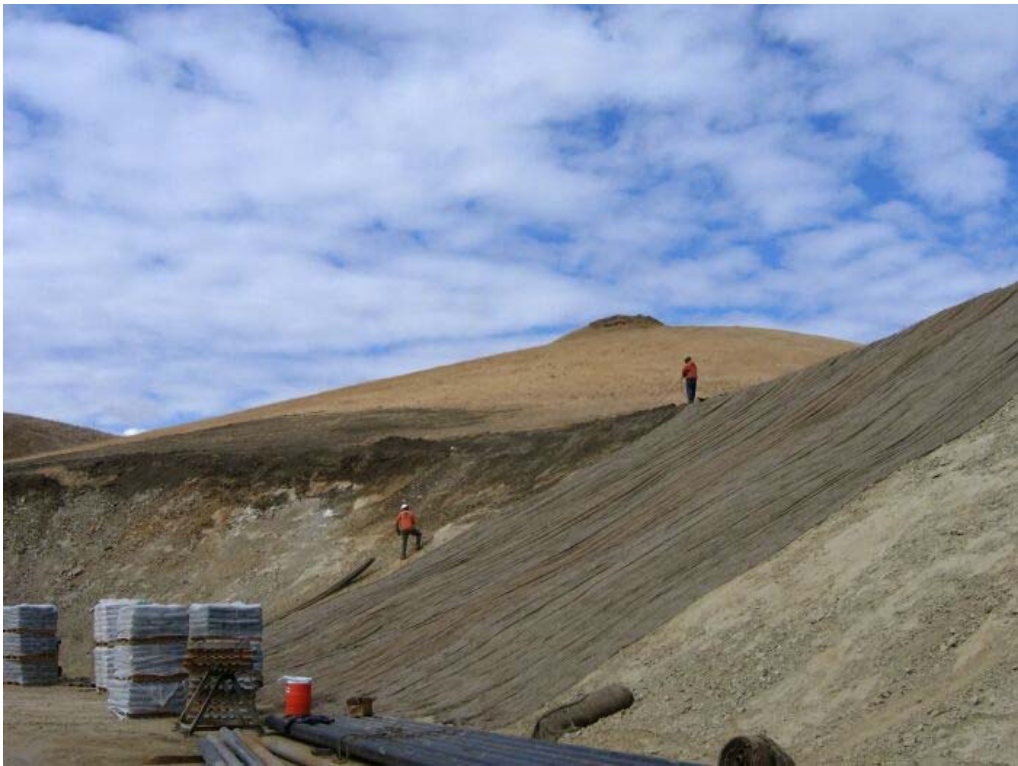
Figure 3 – Erosion controls (jute matting) being installed at well site S-2, October 5, 2006.
