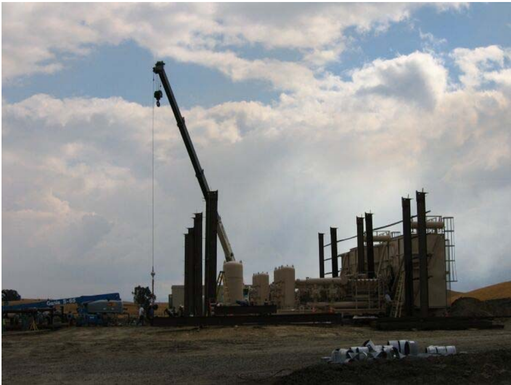
Figure 4 – Compressor building being erected at the Compressor Station, October 5, 2006.
