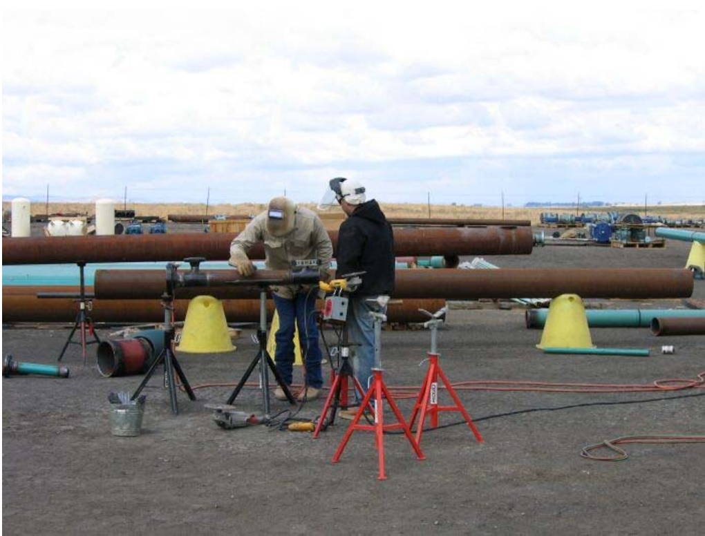
Figure 5 – Crews working on pipe fabrication at the Compressor Station, October 5, 2006.
