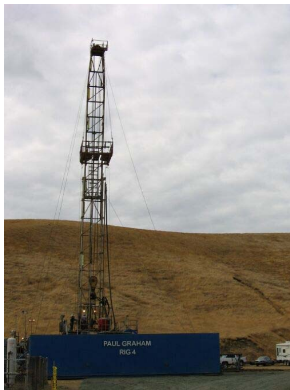
Figure 2 – Drill rig at well site S-2, October 5, 2006.
