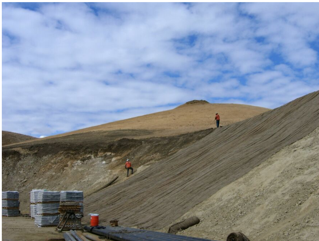
Figure 4-11. Erosion Controls Being Installed at Well Site S-2, 10-05-06
