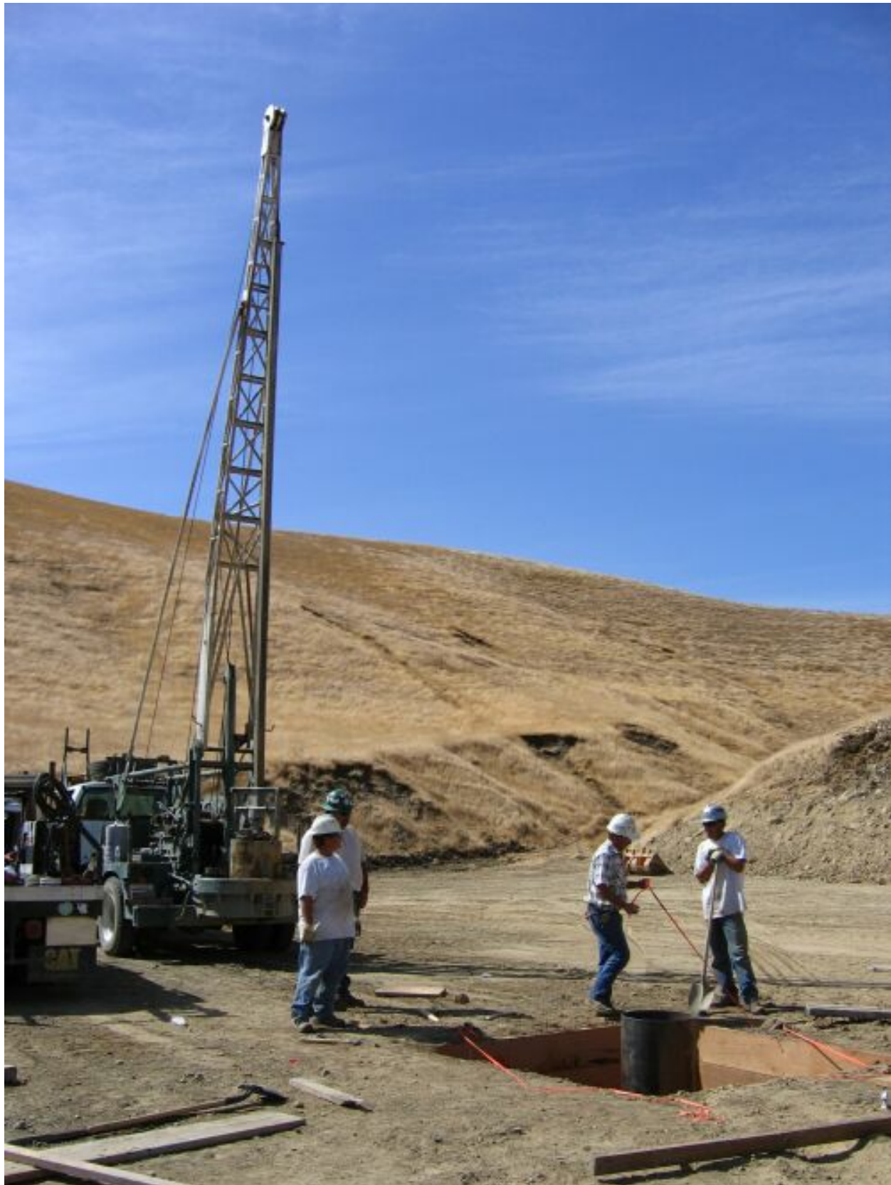
Figure 4-9. Small Drill Rig at Well Site S-2, 9-19-06.
