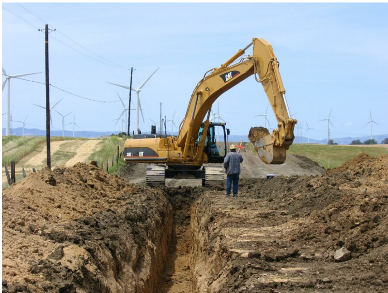
Figure 3-2. Excavating of Pipeline Trench, 5-26-06
