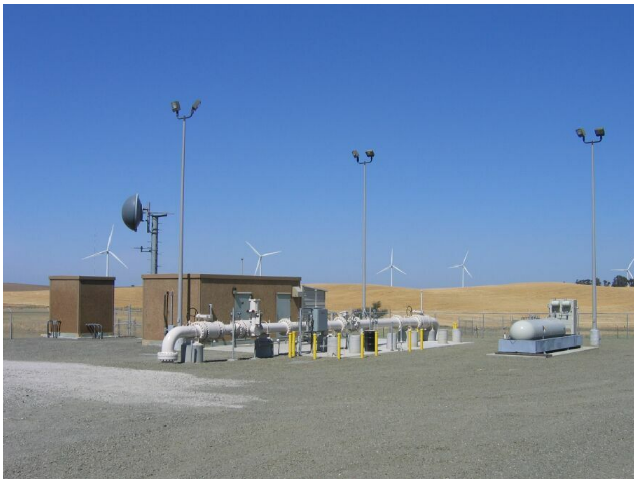
Figure 5-2. Metering Station Work Complete, 7-09-09
