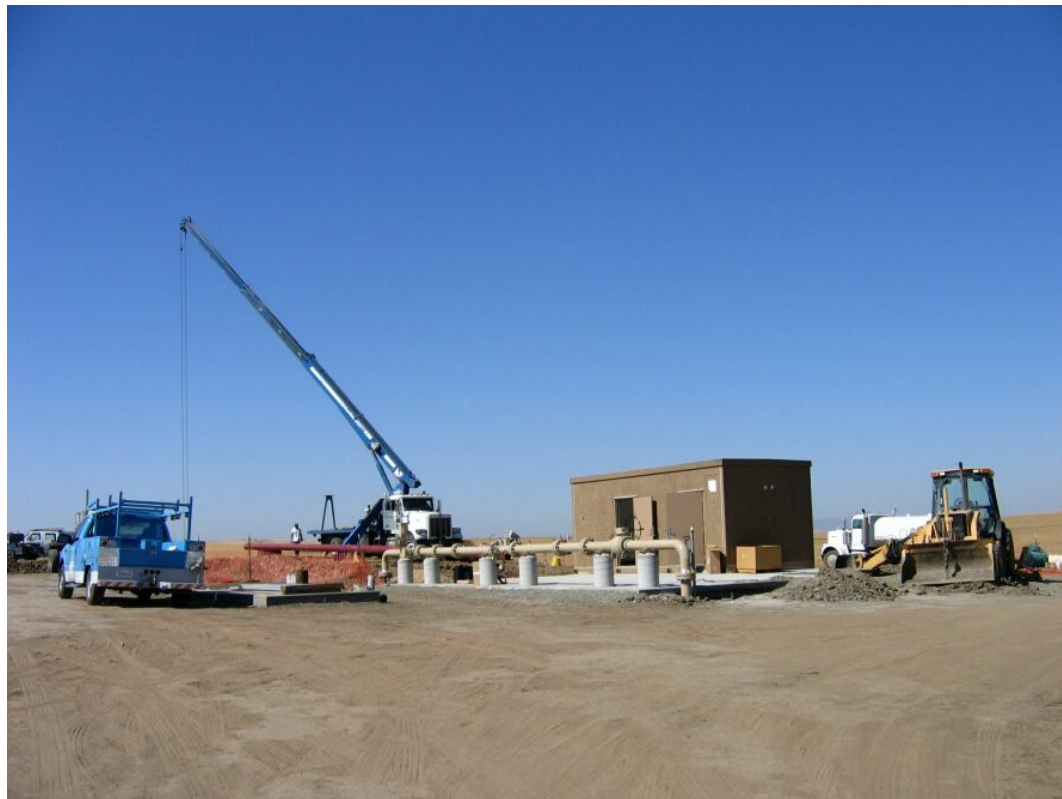
Figure 2-3. Metering Station Construction, 10-12-06
