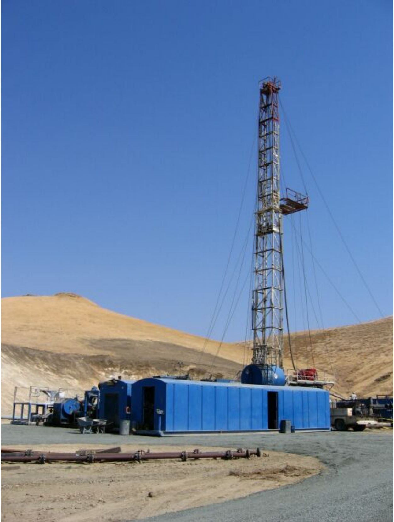
Figure 4-10. Large Drilling Rig at Well Site S-2, 9-26-06
