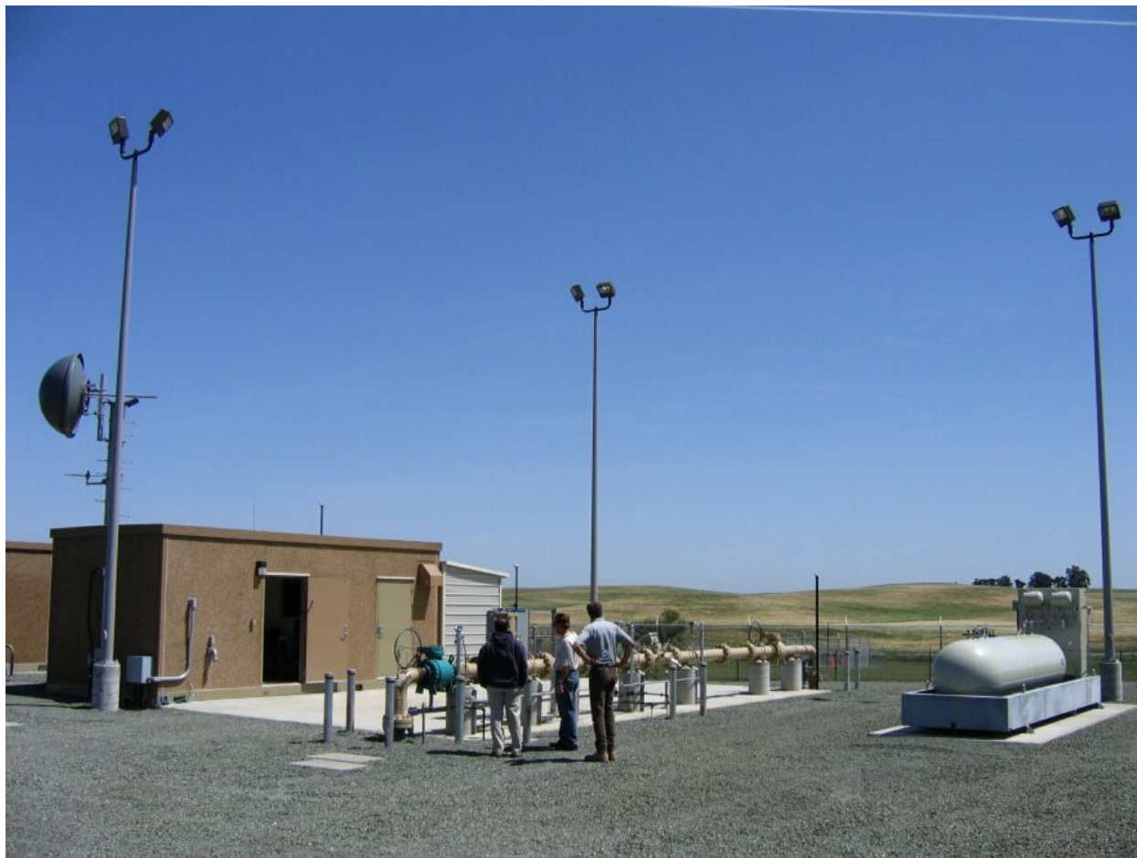
Figure 2-4. Completed Metering Station, 4-26-07
