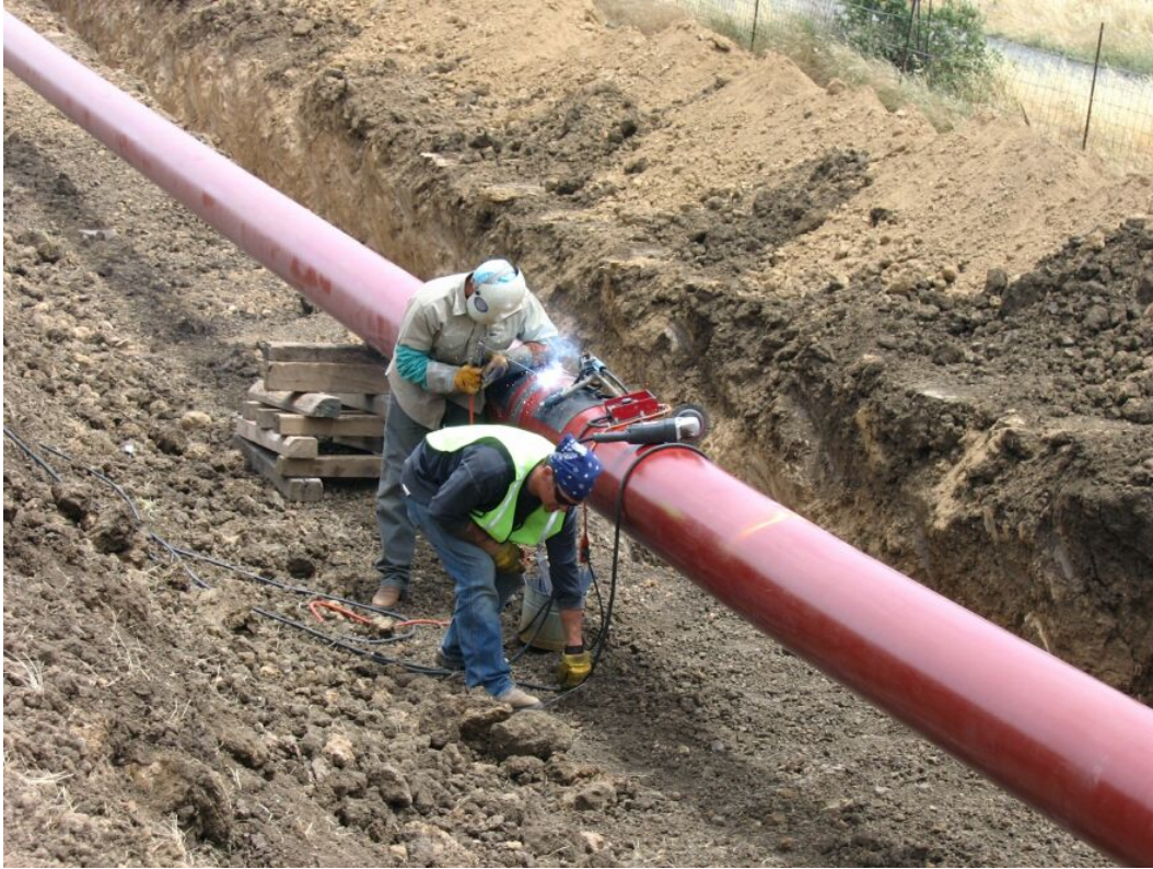
Figure 3-3. Crews Welding Pipe, 6-01-06
