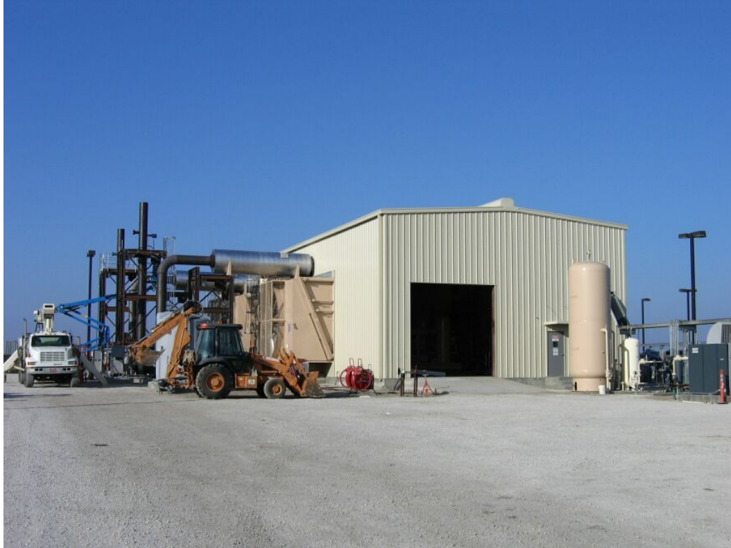
Figure 4-4. Compressor Station Building, 1-23-07
