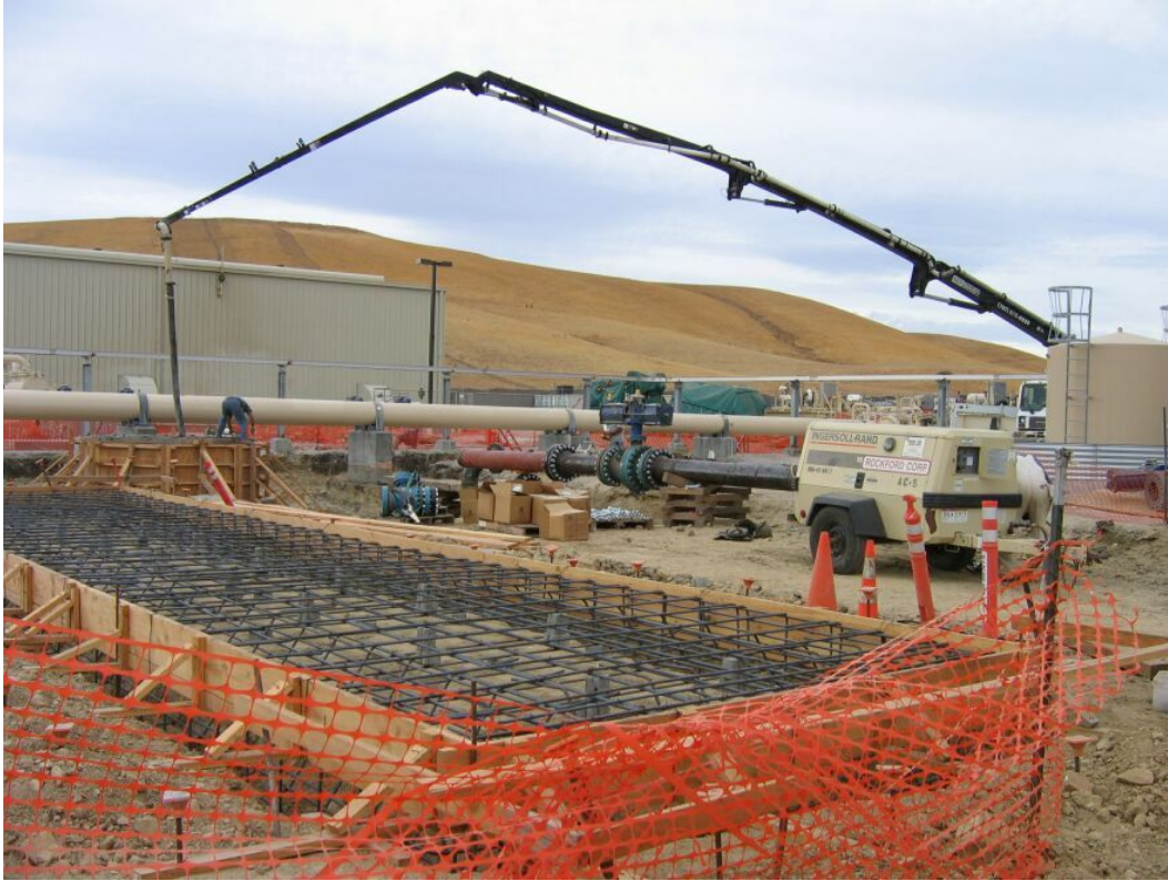
Figure 5-13. Foundation Work at Compressor Station, 10-03-08
