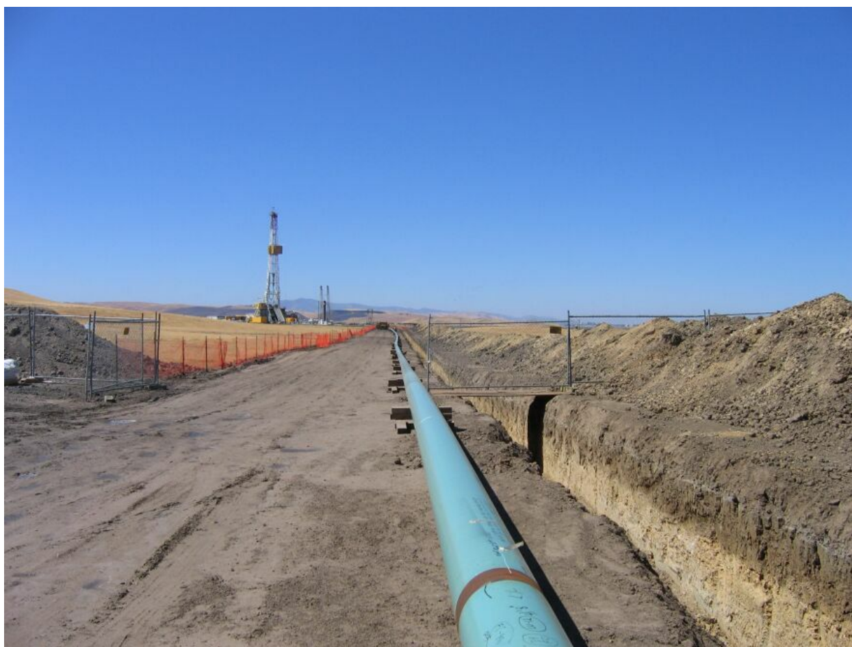
Figure 5-8. Pipeline Installation Between Compressor Station and Well Site 21, 8-08-08.
