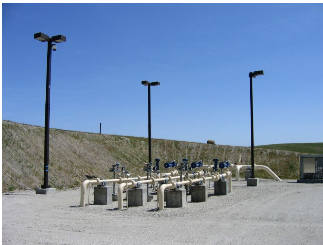
Figure 4-12. Well Site S-2, 4-26-07
