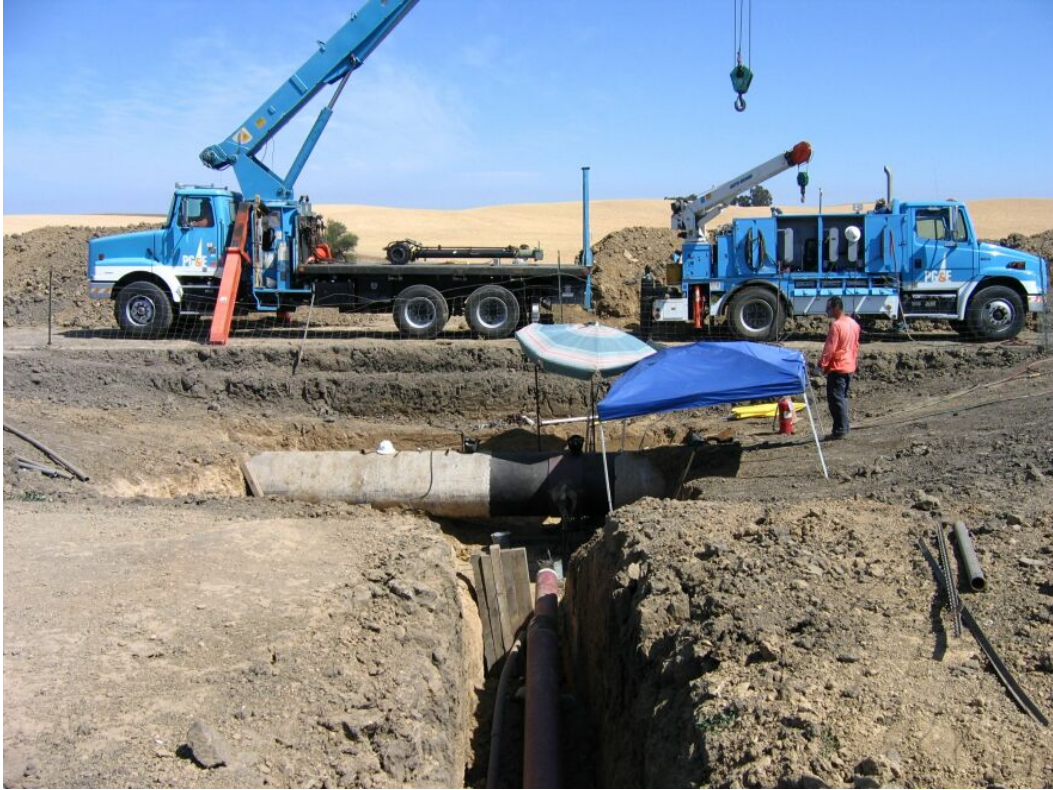
Figure 2-2. PG&E crews working at Metering Station, 9-19-06
