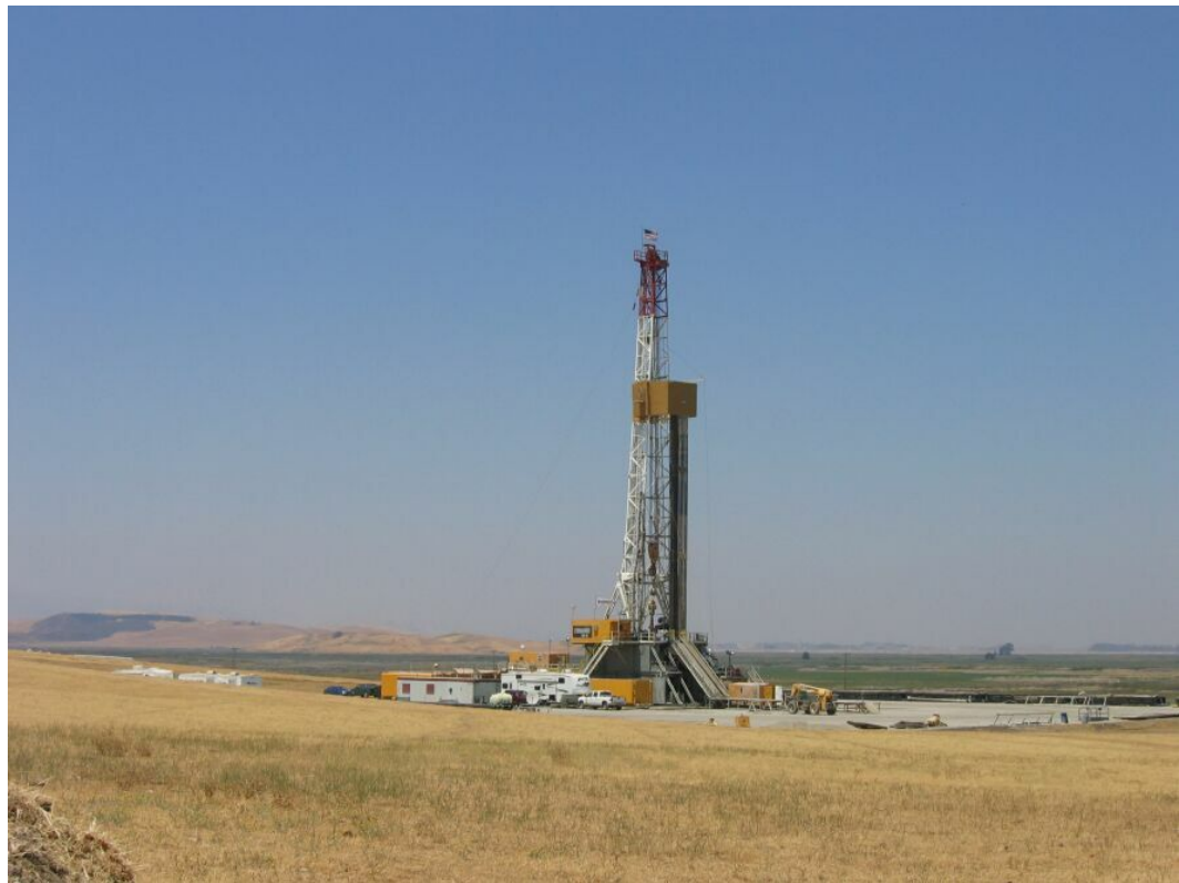
Figure 5-5. Drill Rig Set-up at Well Site 21, 7-18-09
