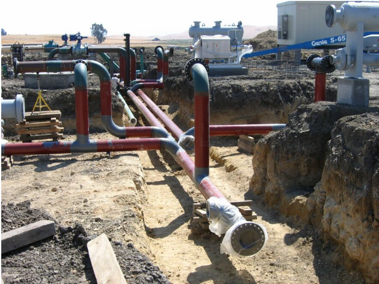
Figure 4-3. Piping Work at Compressor Station, 9-21-06.
