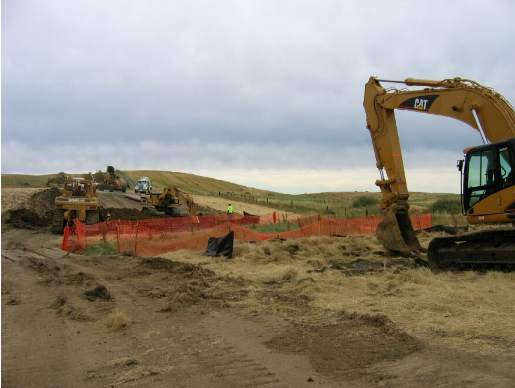
Figure 3-5. Excavating Bore Pits at Drainage, 6-01-06
