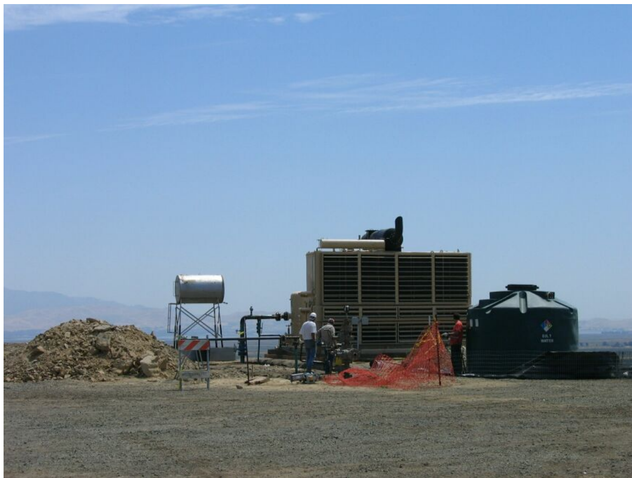
Figure 4-13. Temporary Compressor Installed at Well Site S-10, 7-21-06
