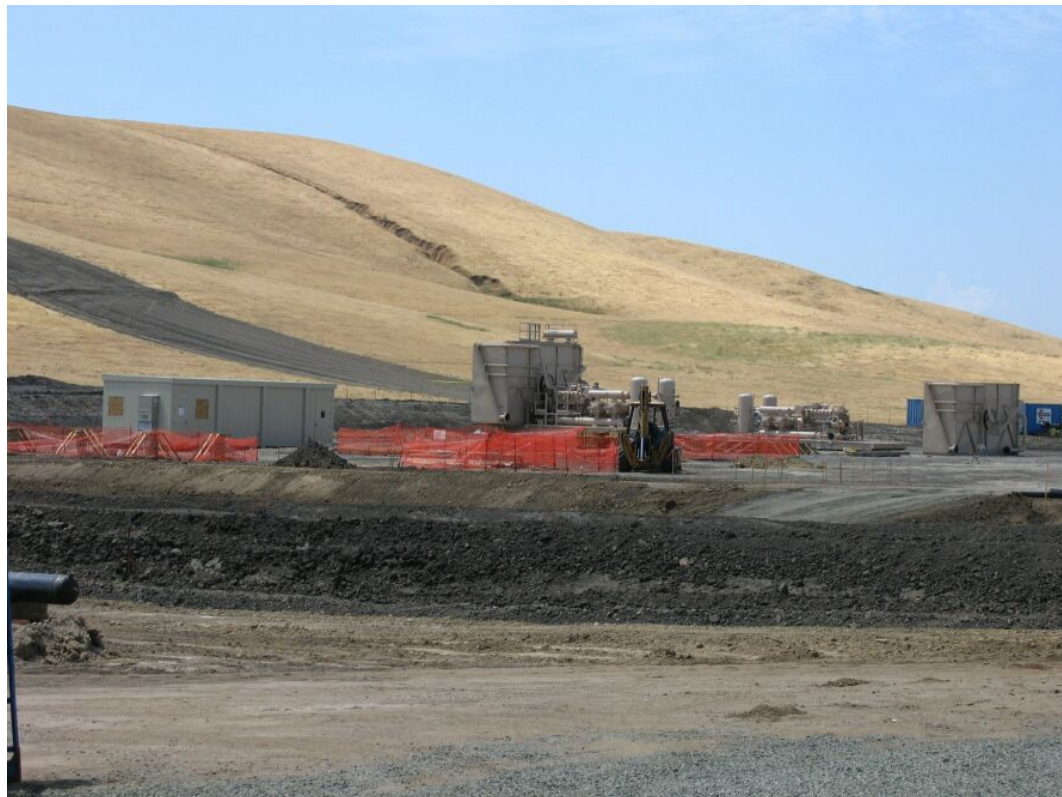
Figure 4-2. Compressors Delivered to Compressor Station Site, 7-21-06
