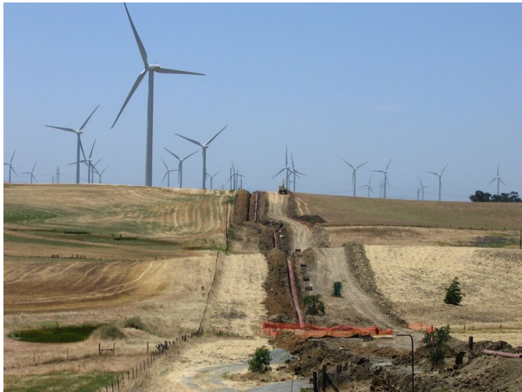
Figure 3-4. Trench ROW Looking West, 6-09-06
