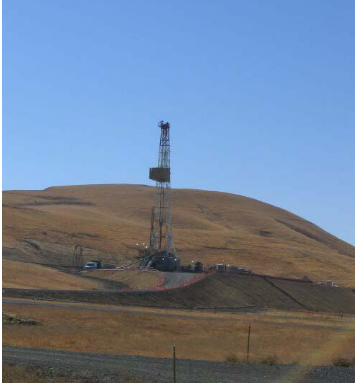
Figure 5-6. Drill Rig Set-up at Well Site 23, 9-12-08
