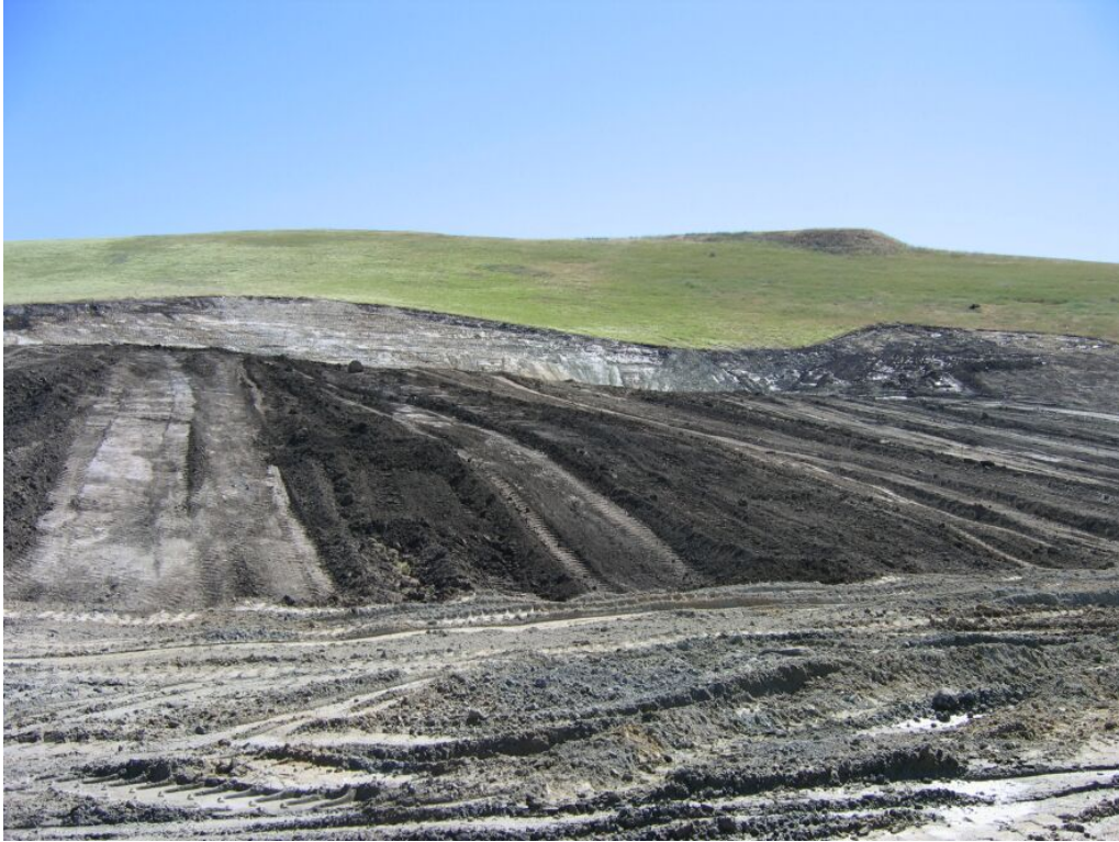
Figure 3 – Well pad grading work at WS-23, May 16, 2008.
