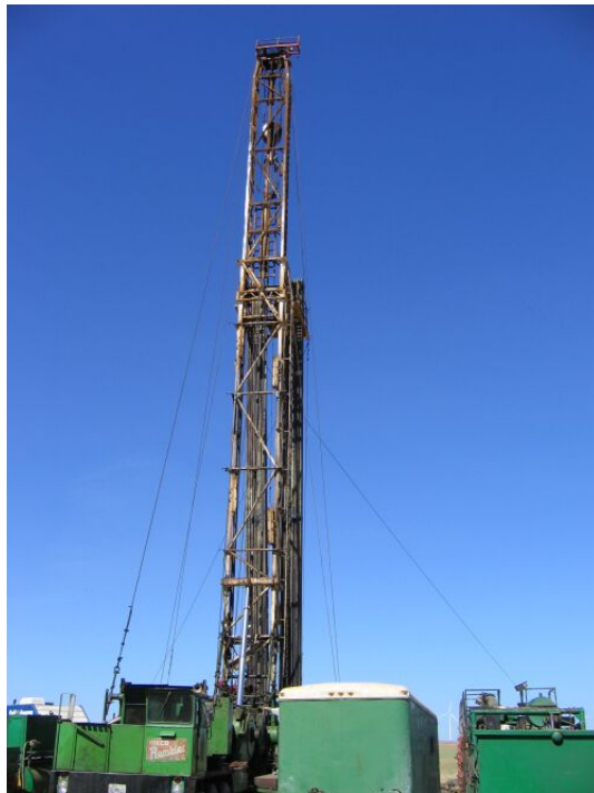
Figure 4 – Workover rig set up at Well L6, May 16, 2008.
