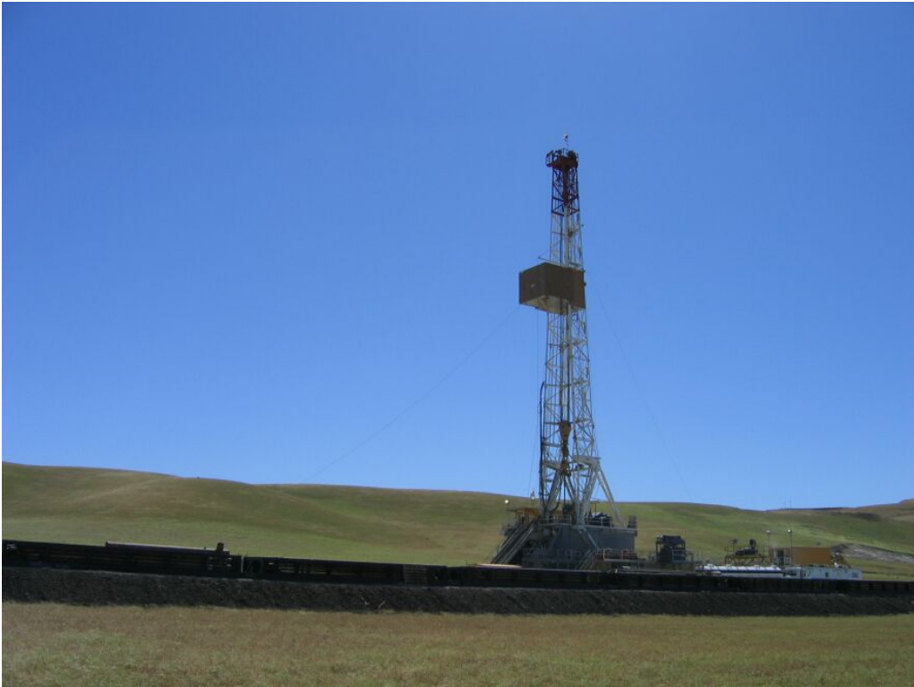
Figure 1 – Drill rig set up at WS-22, May 16, 2008.
