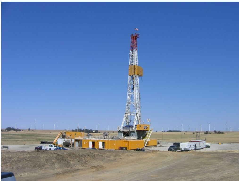
Figure 1 – Drilling operations at WS 22-9 at Well Site 22, May 21, 2008.
