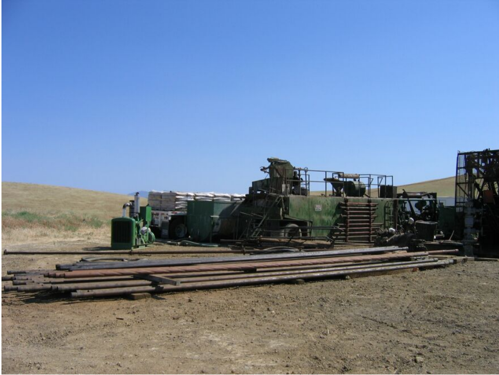
Figure 3 – Workover equipment at Well L6, May 21, 2008.
