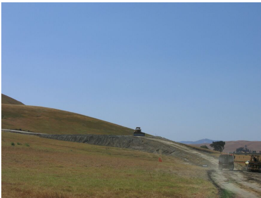
Figure 2 – Crews building up well pad at WS-23, May 21, 2008.
