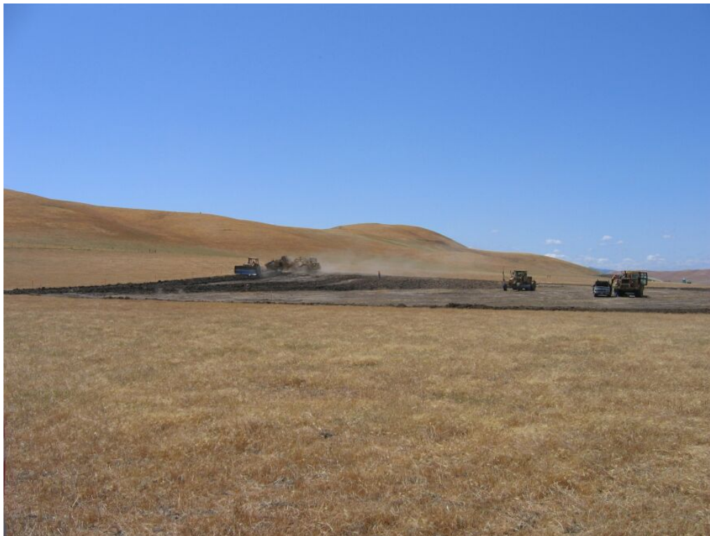
Figure 1 – Clearing and grading of Well Site 21, May 29, 2008.
