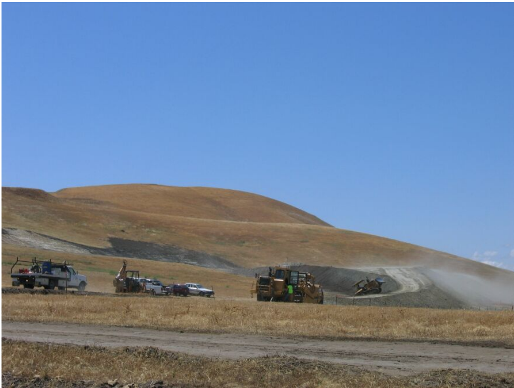
Figure 3 – Crews working on access road to WS-23, May 29, 2008.
