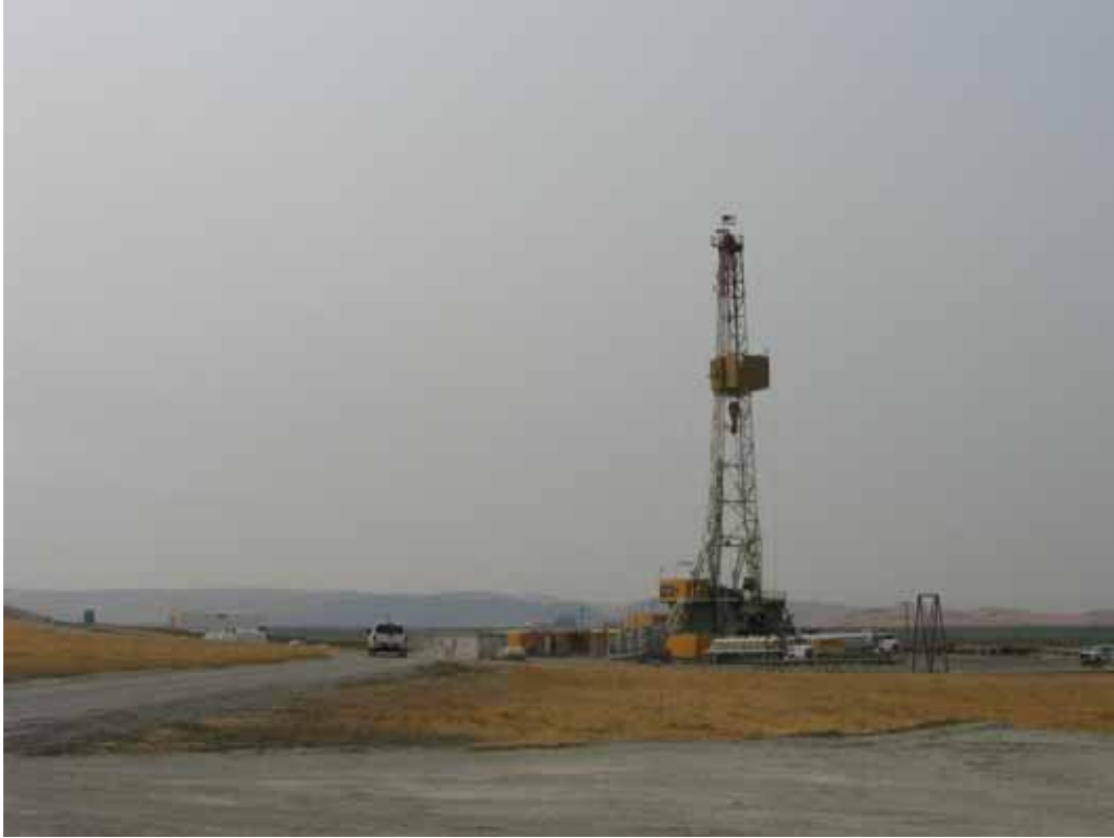
Figure 1 – Drilling rig drilling at WS-22-7 at well pad WS-22, July 10, 2008.
