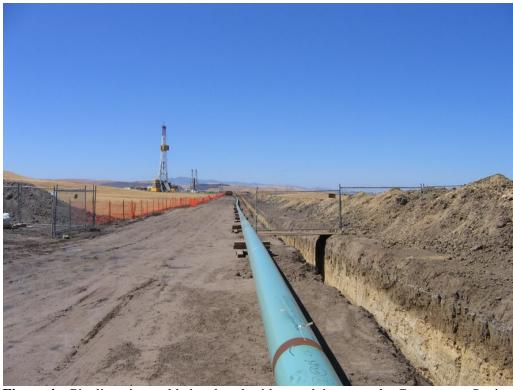
Figure 4 – Pipeline pipe welded and set beside trench between the Compressor Station and WS-21, August 8, 2008.
