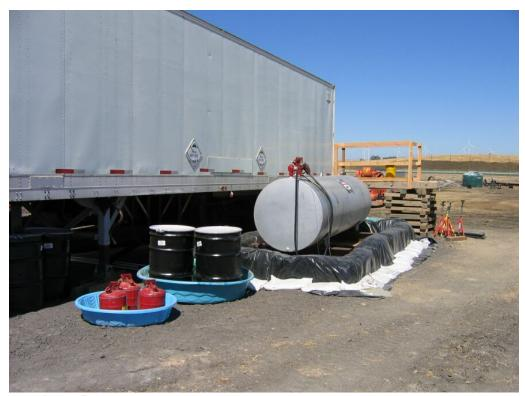
**Figure 5** – Refueling area at Compressor Station with secondary containment, August 8, 2008.
