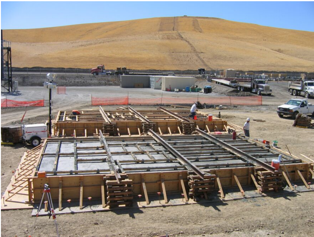
Figure 5 – Foundations for compressors at the Compressor Station, August 28, 2008.
