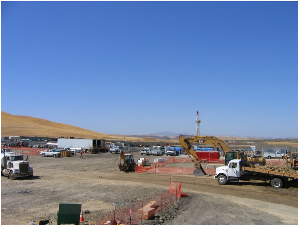
Figure 4 – Compressor Station staging yard, August 28, 2008.
