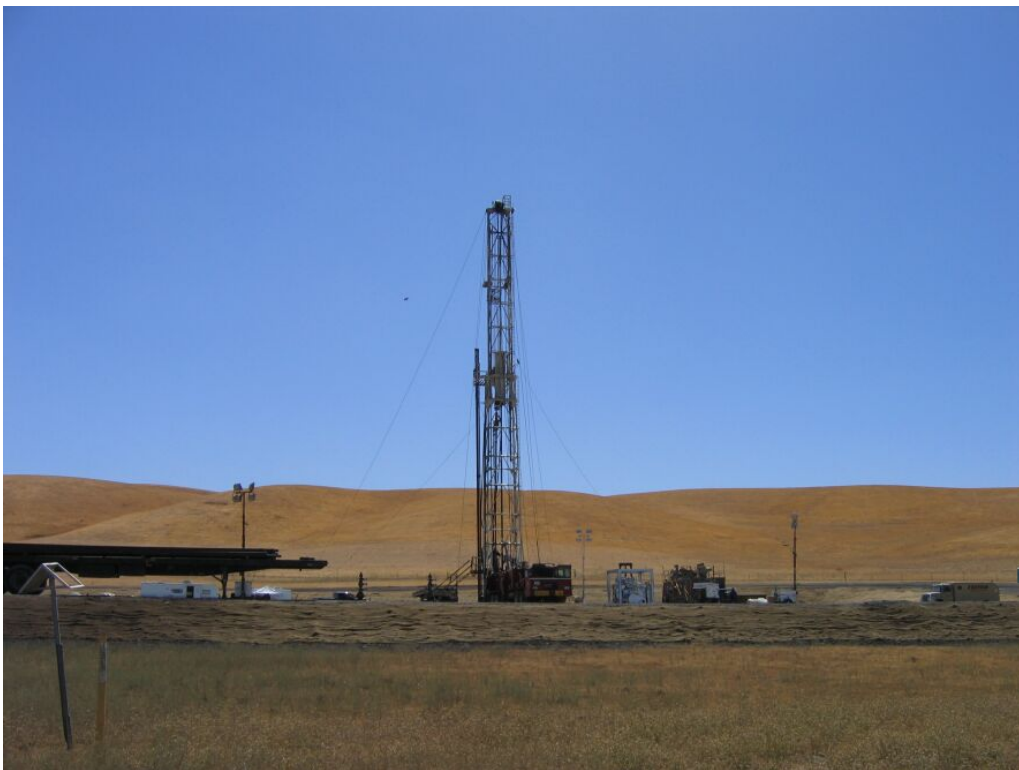
Figure 2 – Workover rig set up at WS-22-9, August 28, 2008.
