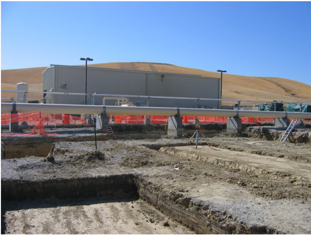
Figure 5 – Excavations for foundations and piping at the Compressor Station, September 12, 2008.
