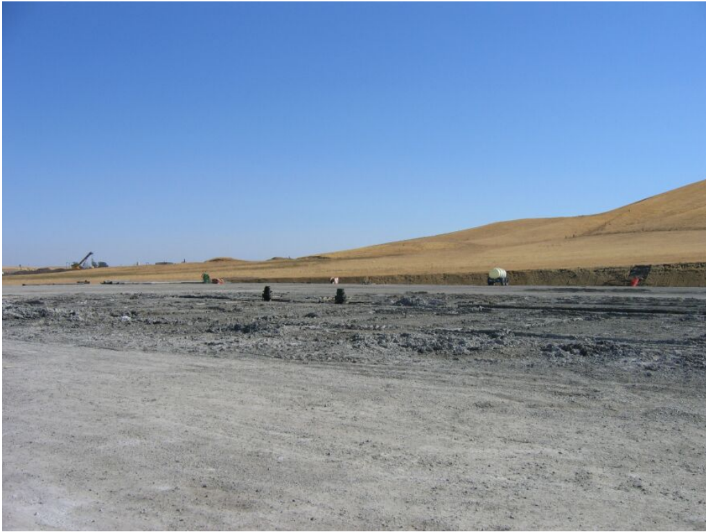
Figure 1 – Drilling completed at WS-21, September 5, 2008.
