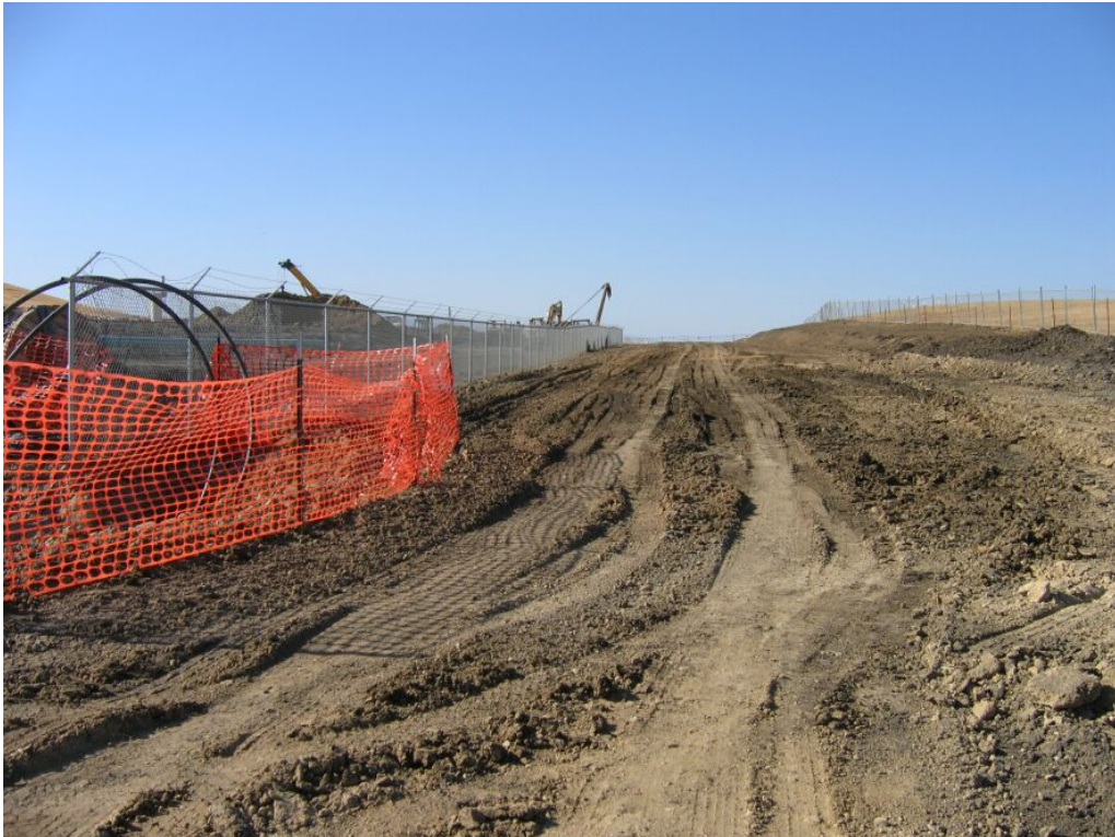
Figure 4 – Pipeline right-of-way on northeast side of Compressor Station, September 5, 2008.
