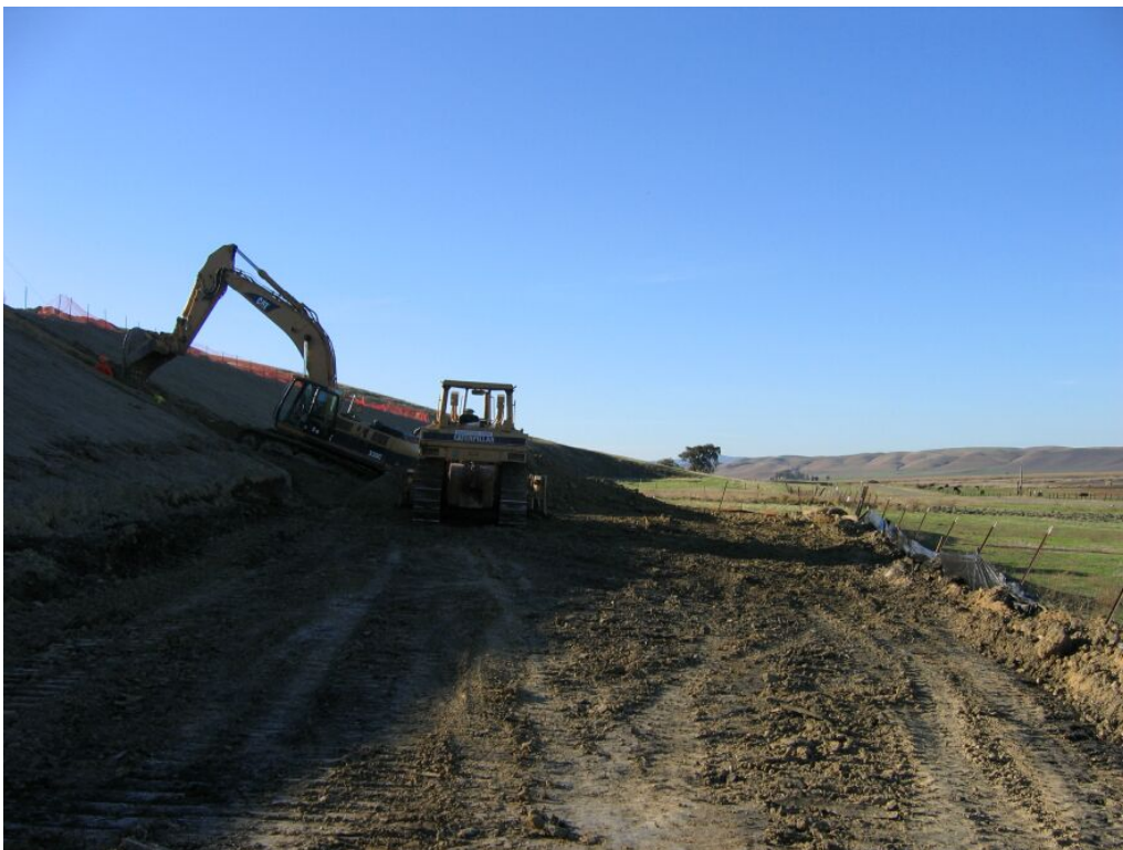
Figure 4 – Excavating pipeline trench on downhill slope of well site 23 (WS-23), November 21, 2008.
