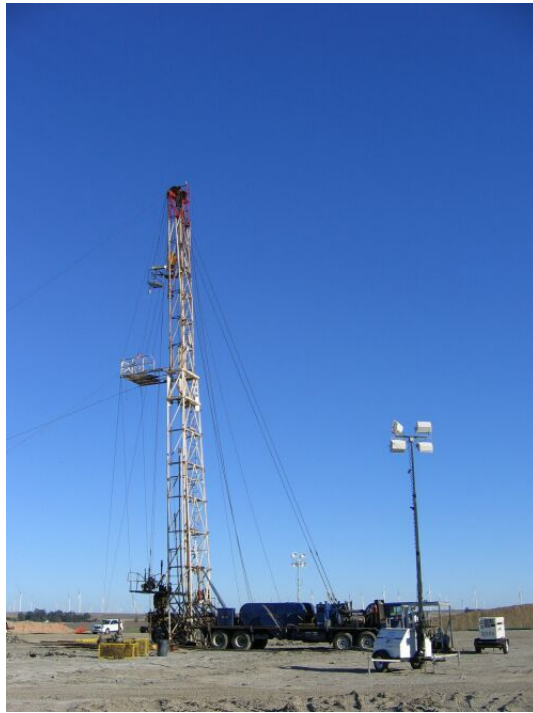
Figure 3 – Workover rig at well site 23 (WS-23), November 21, 2008.
