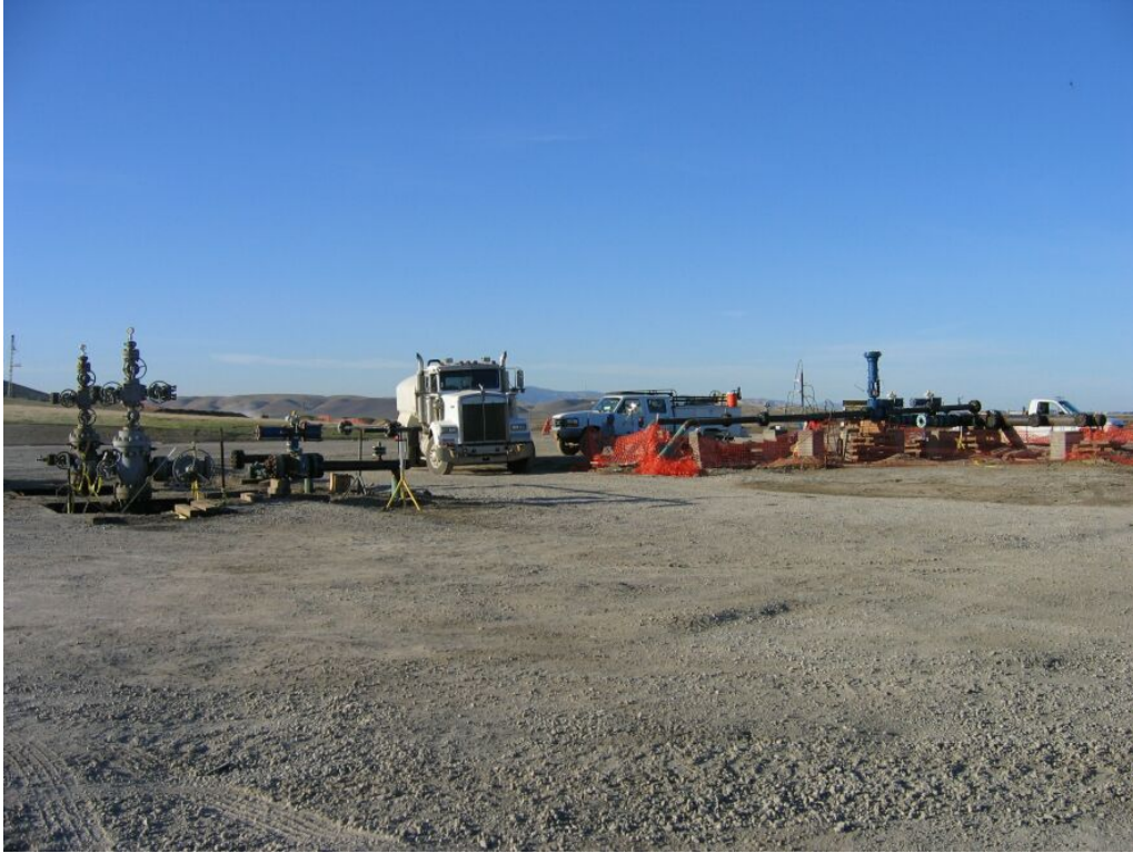
Figure 1 – Crews conducting hydrostatic testing at well site 21 (WS-21), November 21, 2008.
