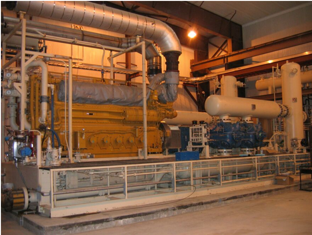
Figure 2 – Inside new compressor building, May 28, 2009.
