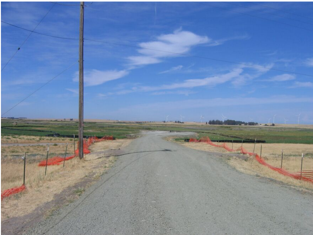
Figure 2 – Wagenet 5 access road and drilling pad, June 25, 2009
