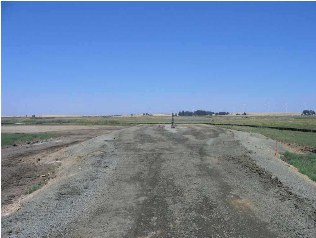
Figure 2 – Well Site 5 well site pad reduced to permanent size, July 9, 2009
