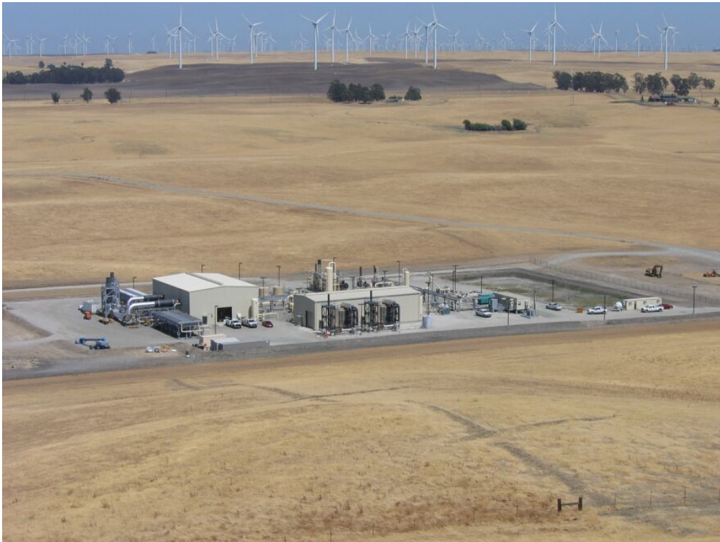
Figure 4 – View of Compressor Station from hillside, July 9, 2009
