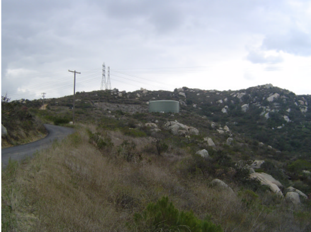
Santee Alt Underground East Side 1.jpg
