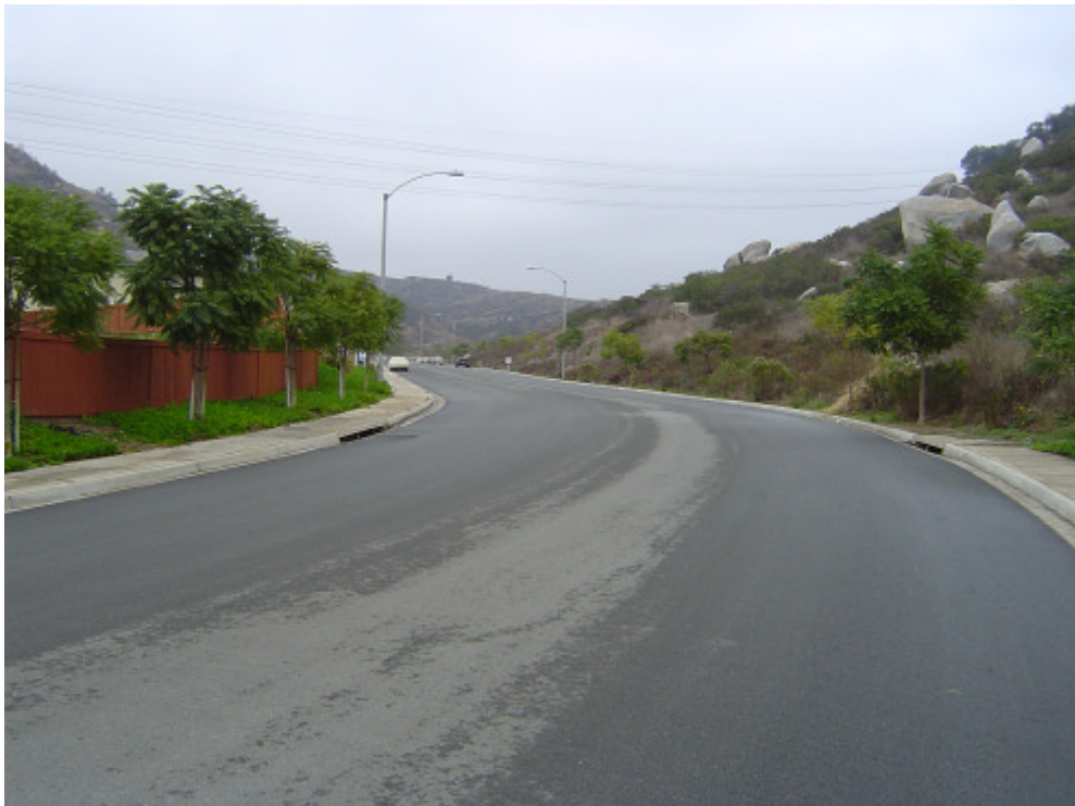
Santee Alt Underground East Side 6.jpg
