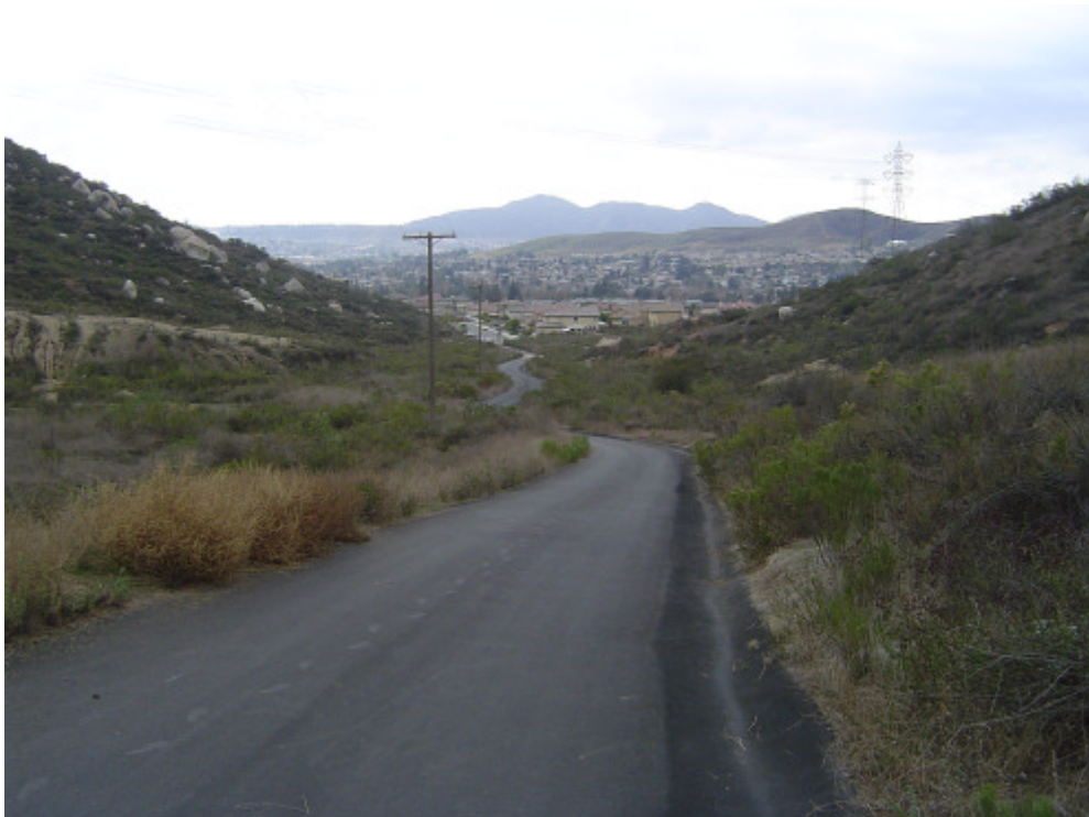
Santee Alt Underground East Side 4.jpg
