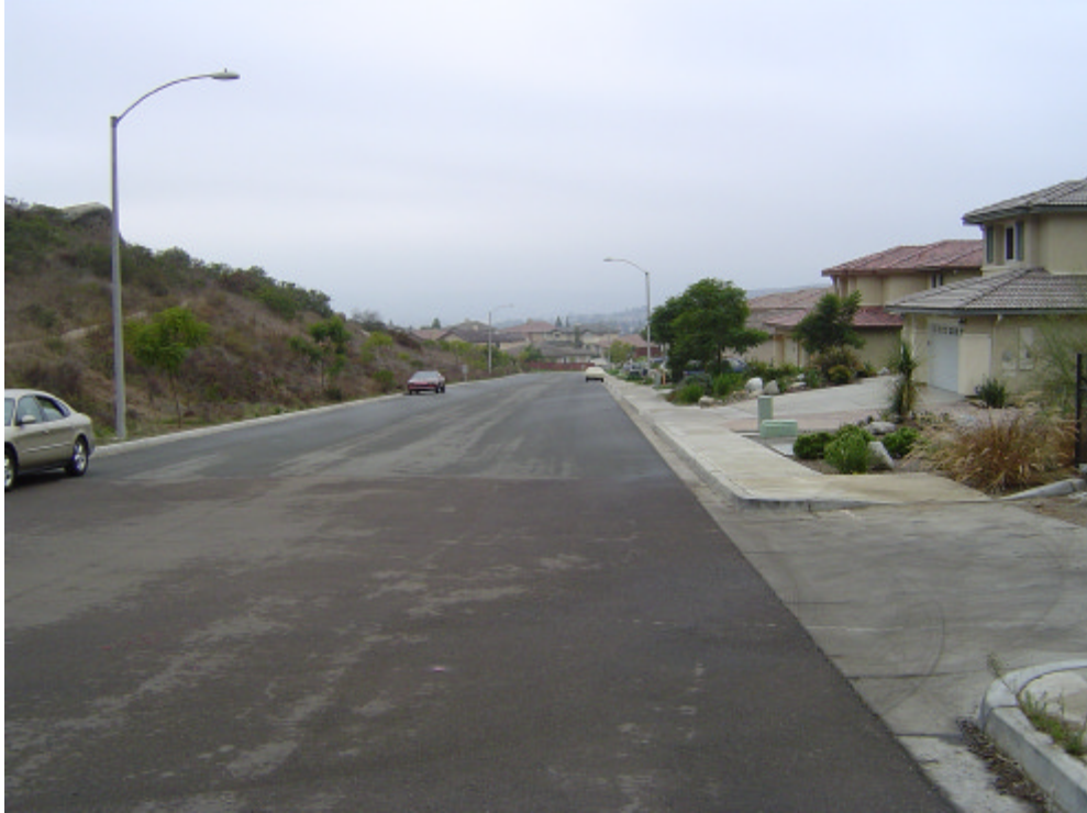
Santee Alt Underground East Side 5.jpg
