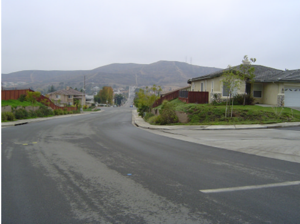
Santee Alt Underground East Side 7.jpg
