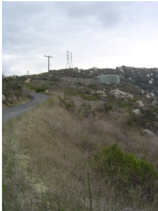
Santee Alt Underground East Side 2.jpg
