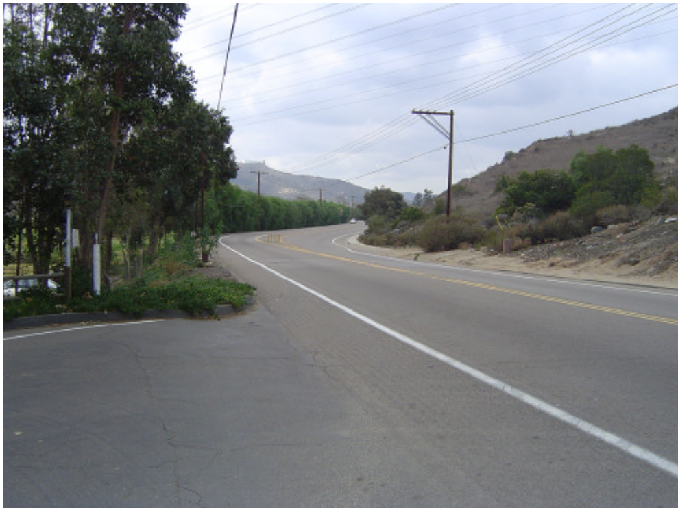
4 Willow Glen Rd & Golf Course Transition Location 4.jpg
