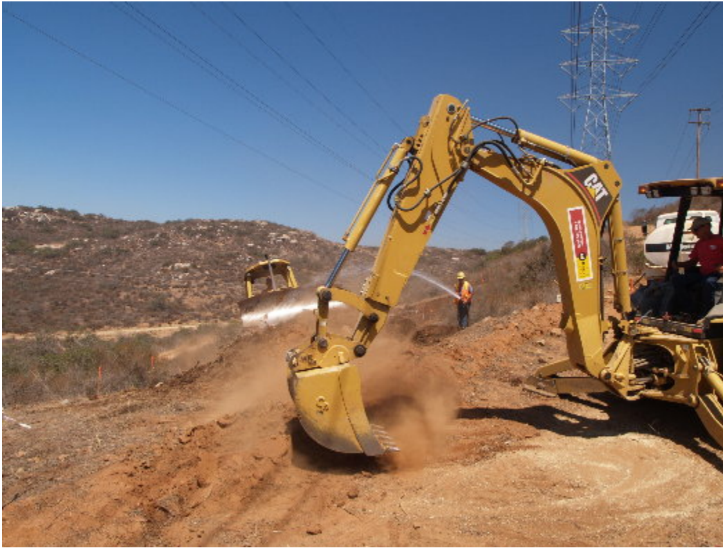
Figure 5 – An operator cut a transition from pad to access road at Site 321.
