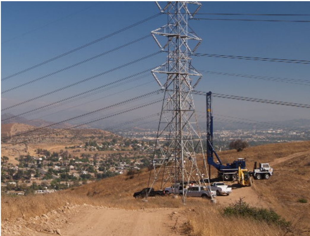
Figure 2 – PAR started boring work for transmission tower foundations at Site 1400.
