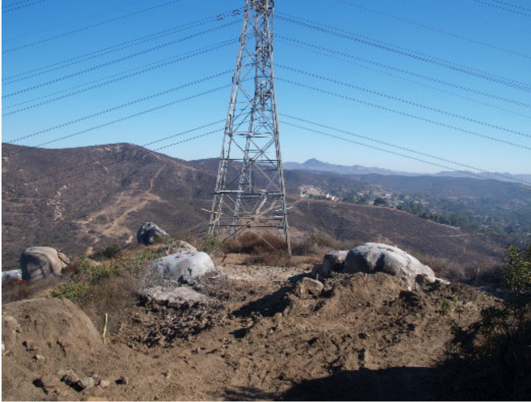
Figure 1 – Site 1300 cleared and holes drilled to prepared for blasting.
