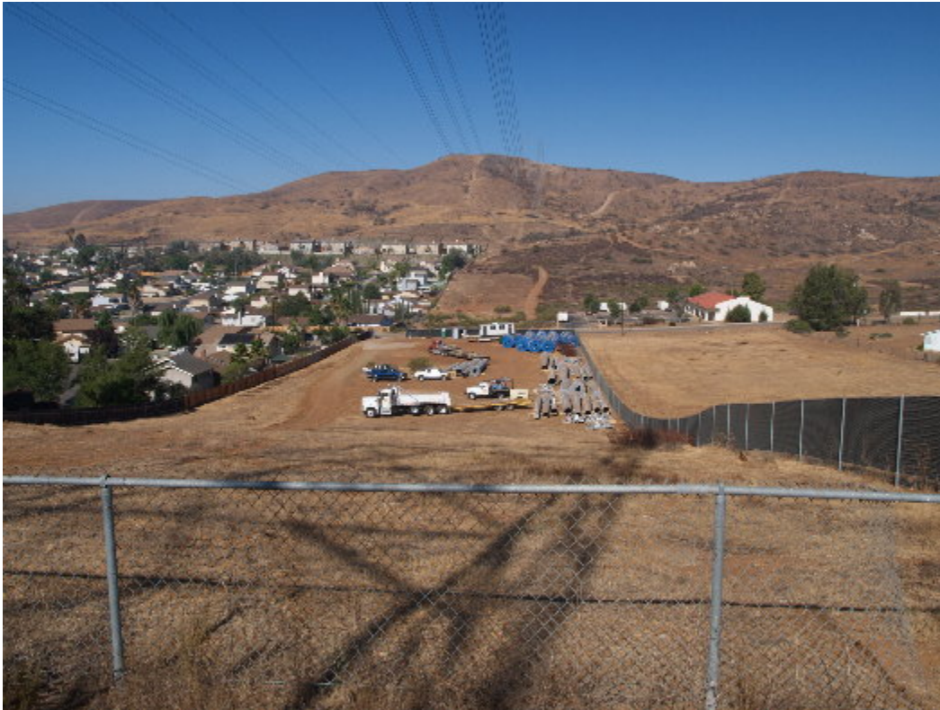
Figure 3 – Laydown site at Summit being used for material storage.
