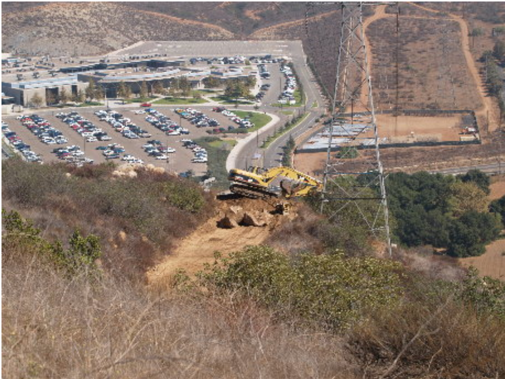
Figure 2 – The operator in the excavator moved boulders off Tower Site 242.
