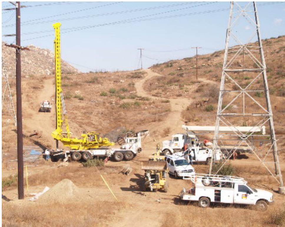
Figure 4 – The drilling crew worked in hard material at Tower Site 842.
