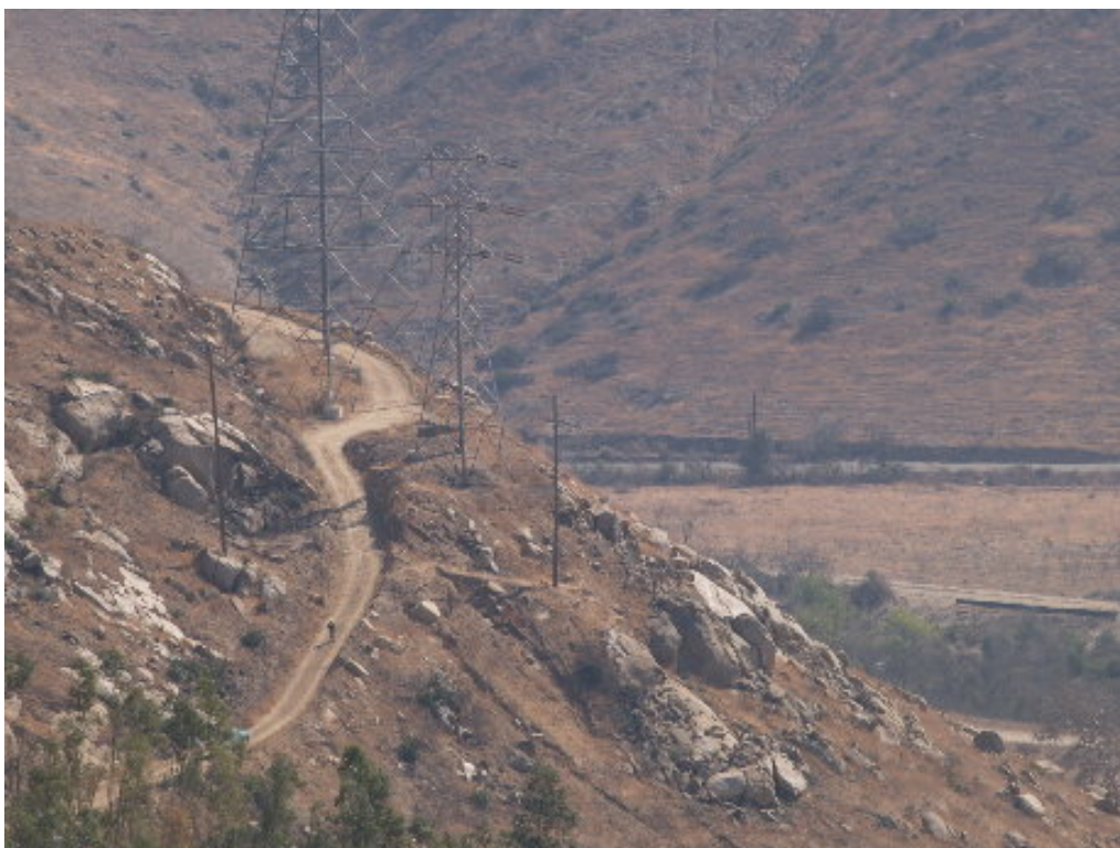
Figure 2 – The construction contractor reviewed engineering changes at Tower Site 1160.
