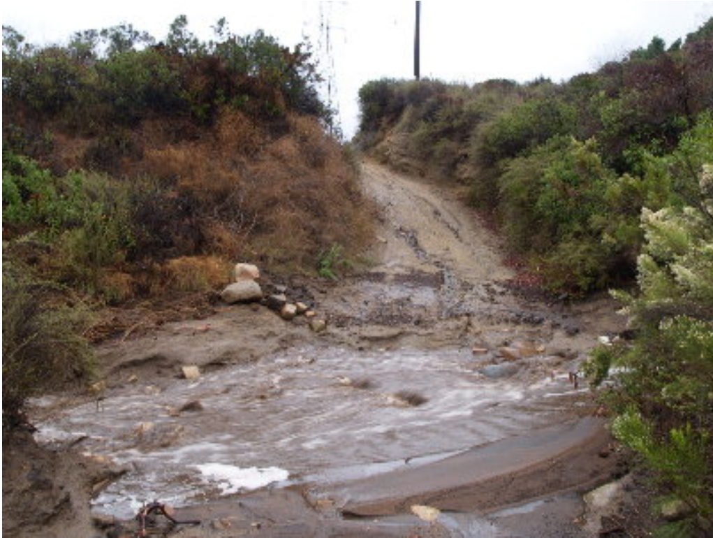
Figure 5 – Both erosion on the access roads and drainage from the surrounding hillsides made access impossible in some areas.
