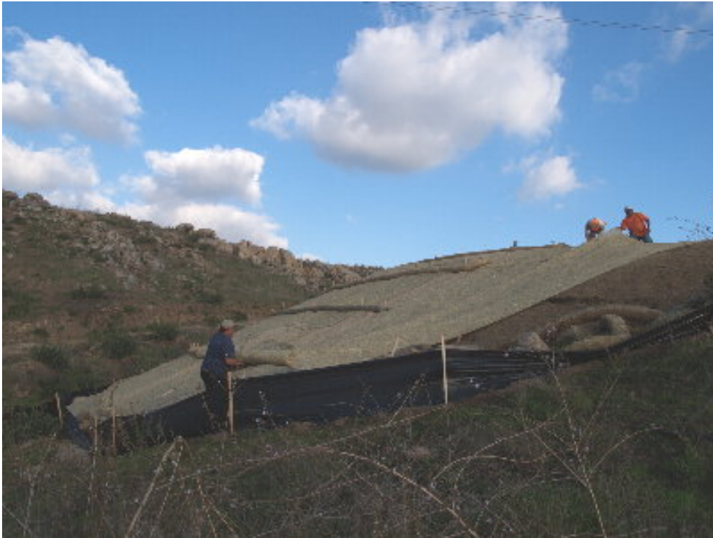
Figure 3 – The Union crew started reseeding and placing straw matting.
