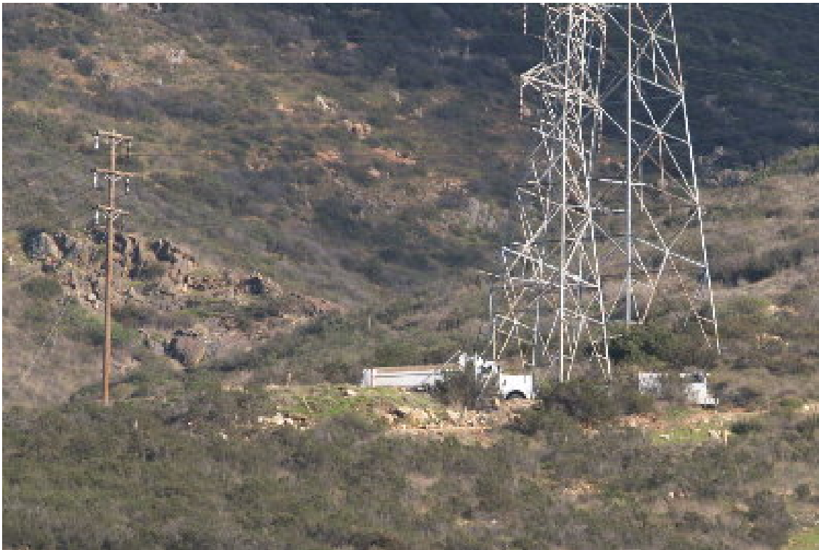
Figure 2 – A mechanic worked on the broken dump truck at Tower Site 151.
