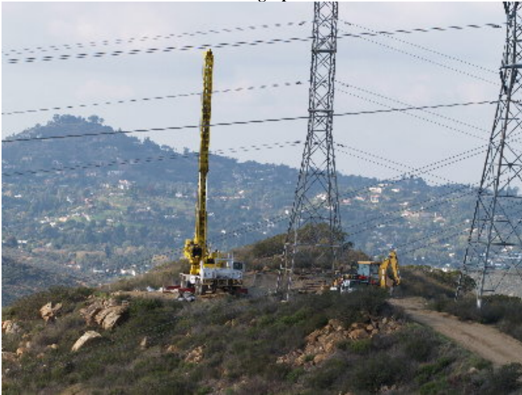
Figure 1 – Drilling continued at Tower Site 221.
