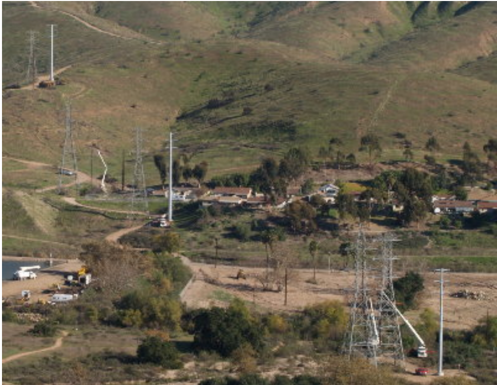
Figure 2 – Support vehicles protected other utilities and the cable during stringing operation.
