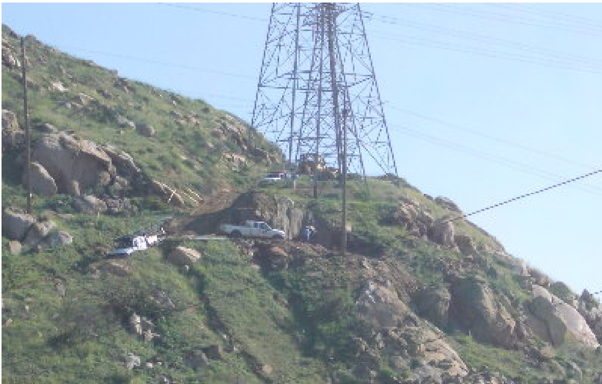
Figure 2 – The concrete crew prepared Tower Site 635c for pouring.
