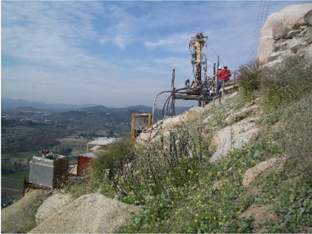
Figure 3 – A crew worked to micro-pile Tower Site 1170 on the steep sidehill.
