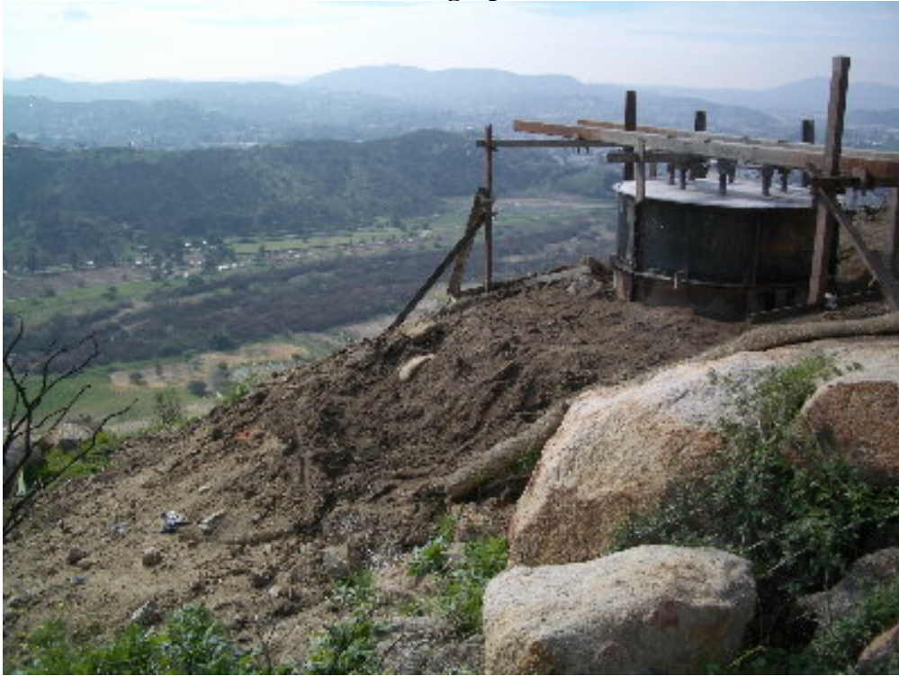
Figure 1 – Loose material at Tower Site 1180 needs to be stabilized prior to the predicted storm.
