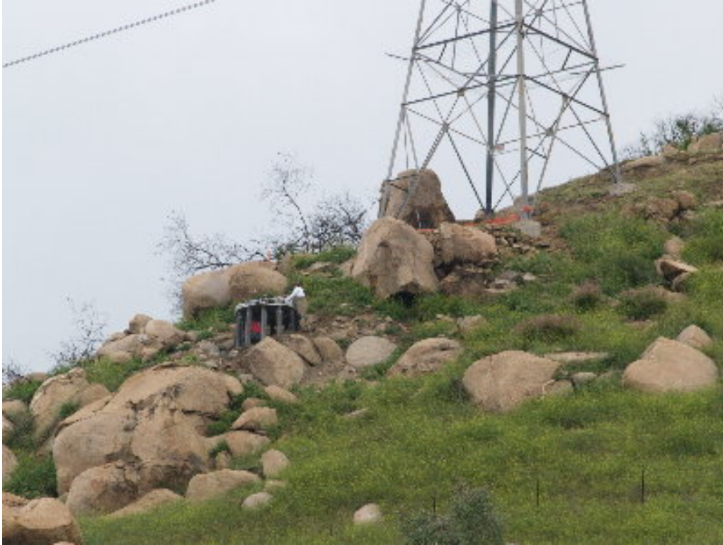
Figure 1 – A testing crew worked to check the micro-piles at Pole Site 1170.
