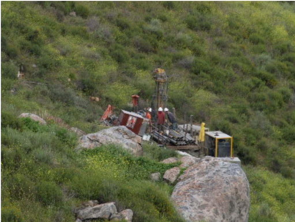
Figure 4 – The micro-pile crew set up at Pole Site 522 and started working.
