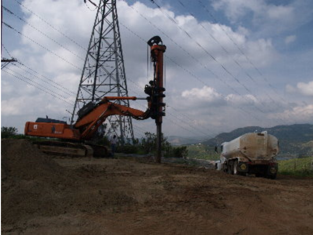
Figure 3 – The drilling at Pole Site C continued during the site visit.
