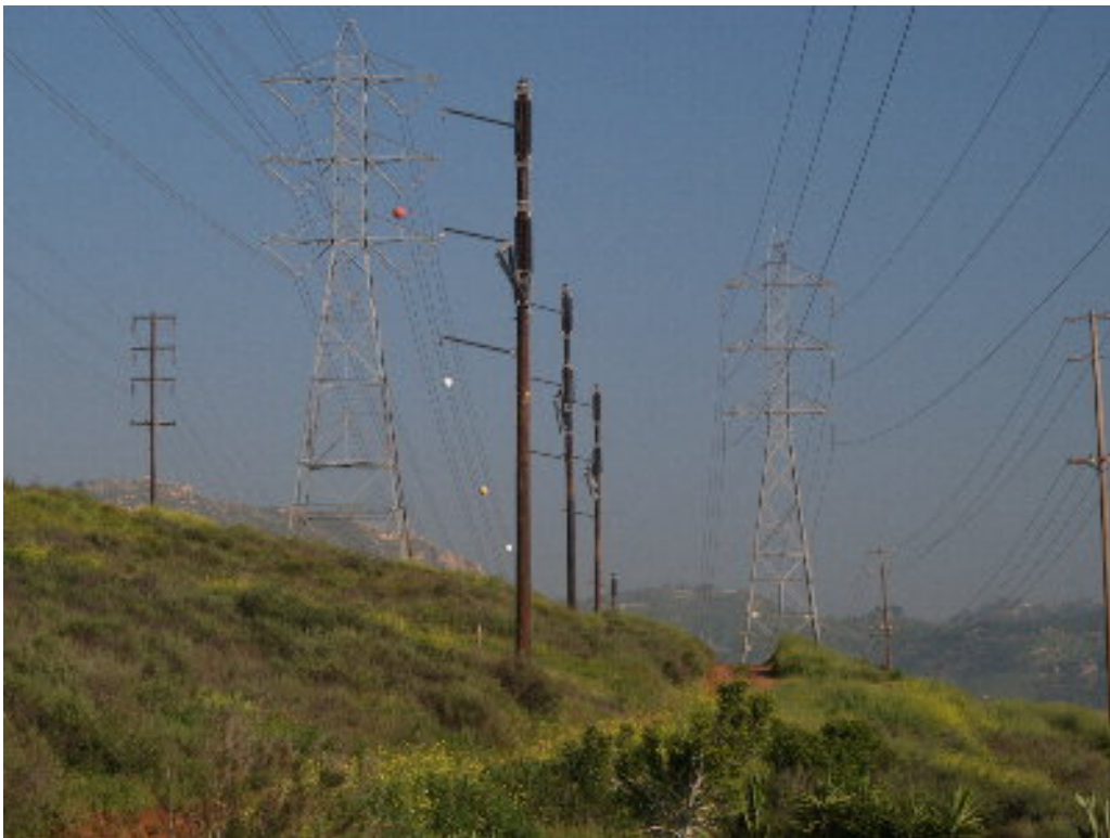
Figure 10 – Five temporary 230 kV wood poles were set during the site visit.
