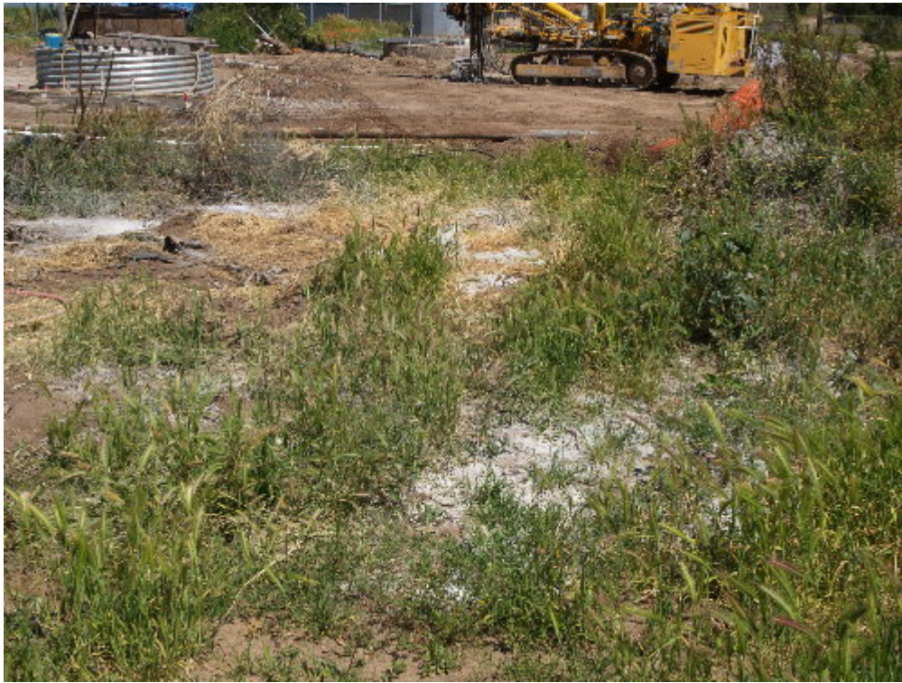
Figure 5 – Grout from the pressure grouting operation spread into the adjacent grasses on the property at Pole Site 1210.
