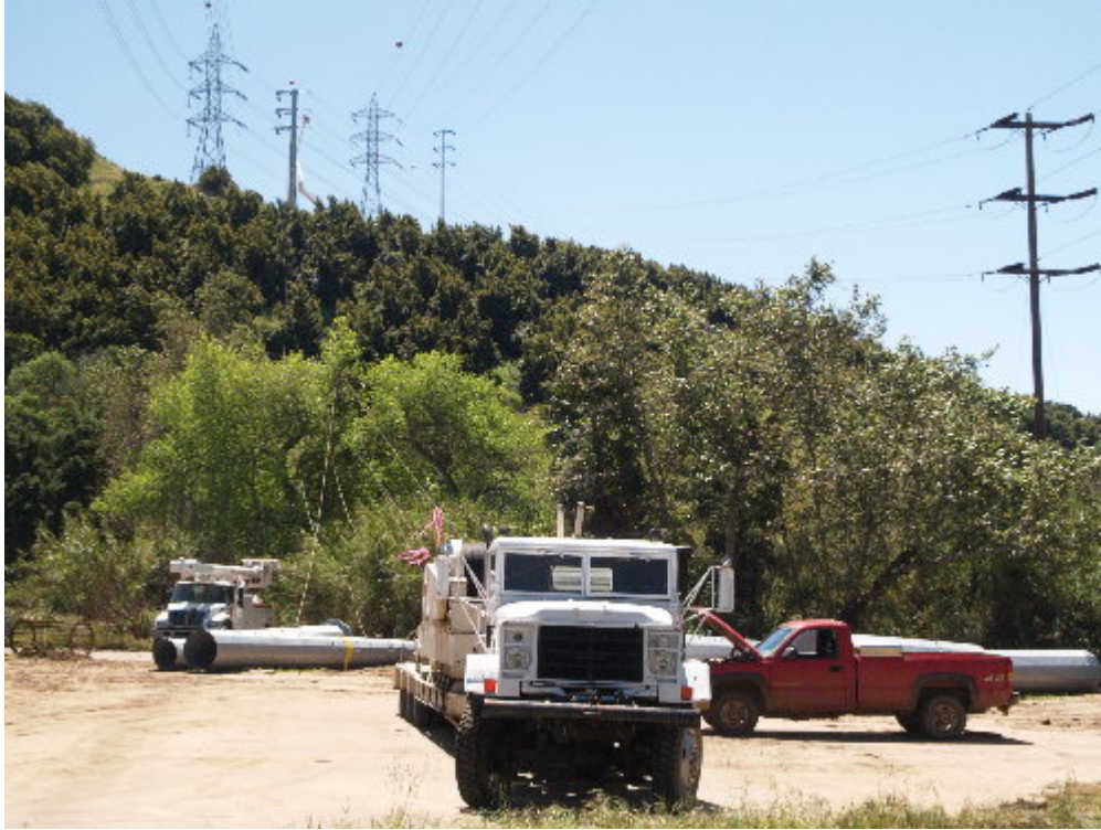
Figure 1 – An SDG&E transmission line crew pulled conductor south of Interstate 8.
