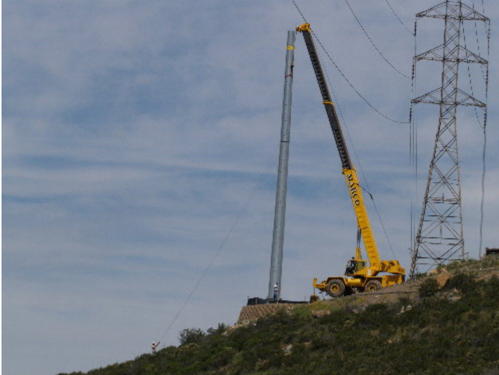
Figure 1 – PAR worked to raise the steel pole sections at Pole Site 181.
