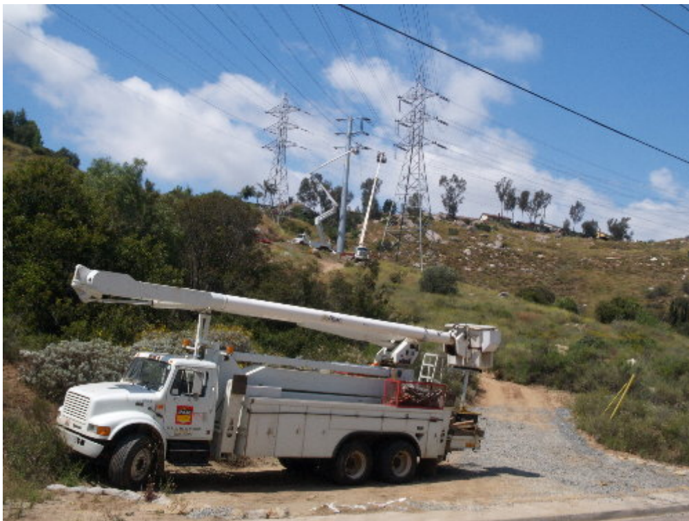
Figure 2 – The PAR crew worked on the conductor at Site 440.
