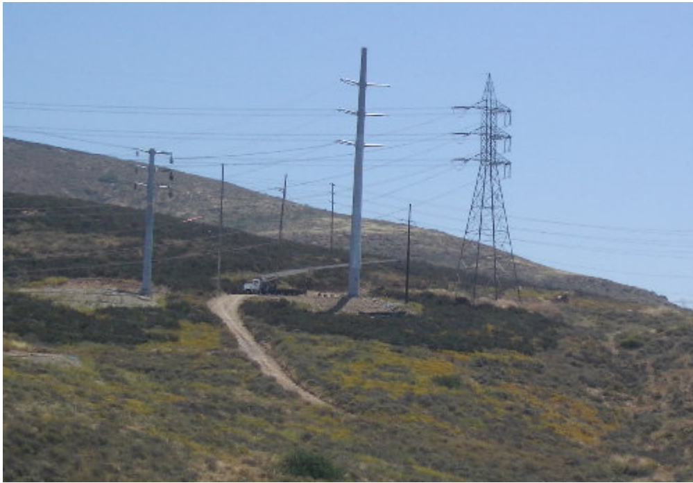
Figure 6 – PAR stringing crew working on the temporary 230 kV system above the Miguel Substation.
