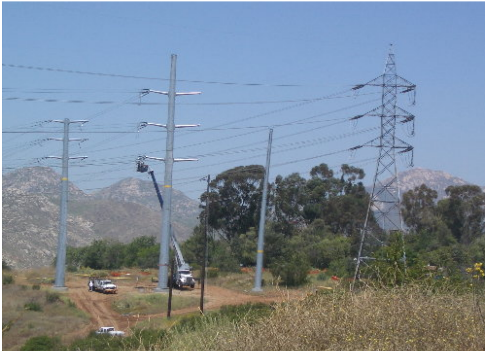
Figure 2 – The Wilson stringing crew installing jumpers above the Los Coches Substation.
