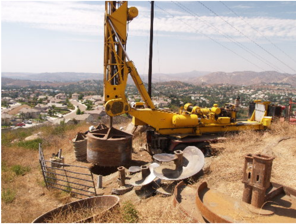
Figure 3 – Tri-State Drilling worked at Steel Pole 581 excavating the foundation.
