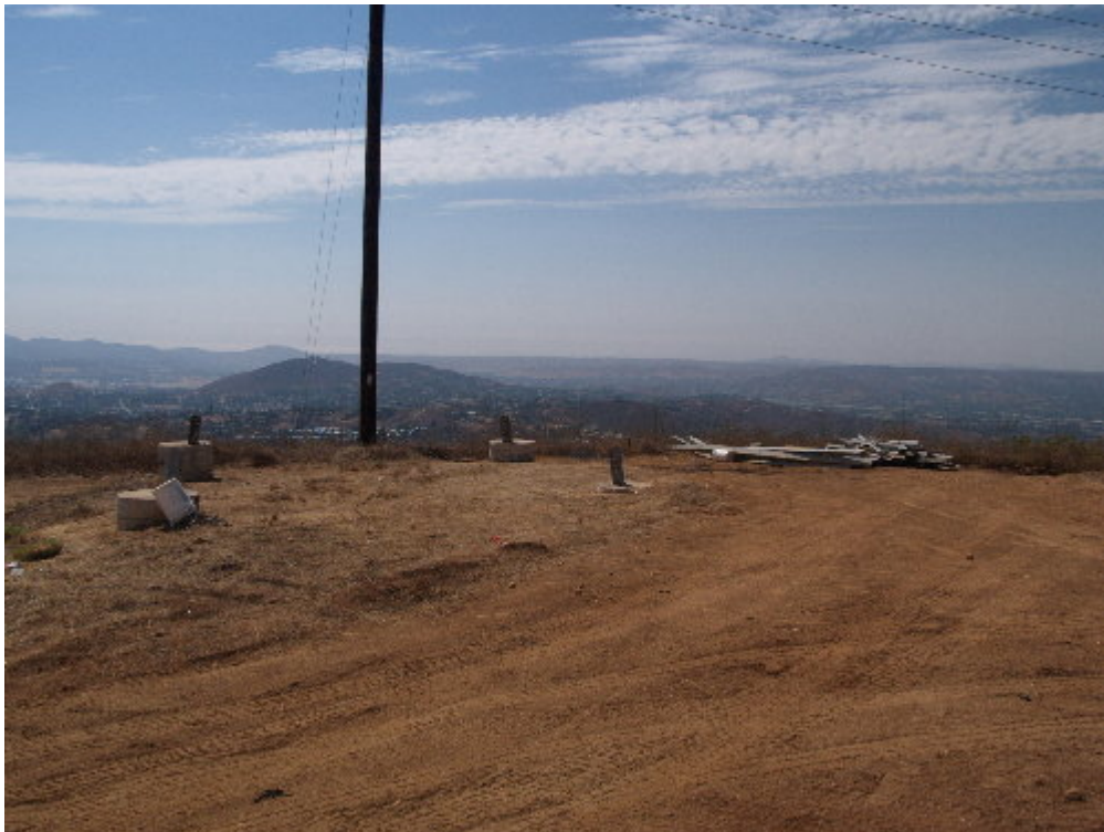
Figure 2 – Wilson Construction has dismantled several towers in preparation for drilling.
