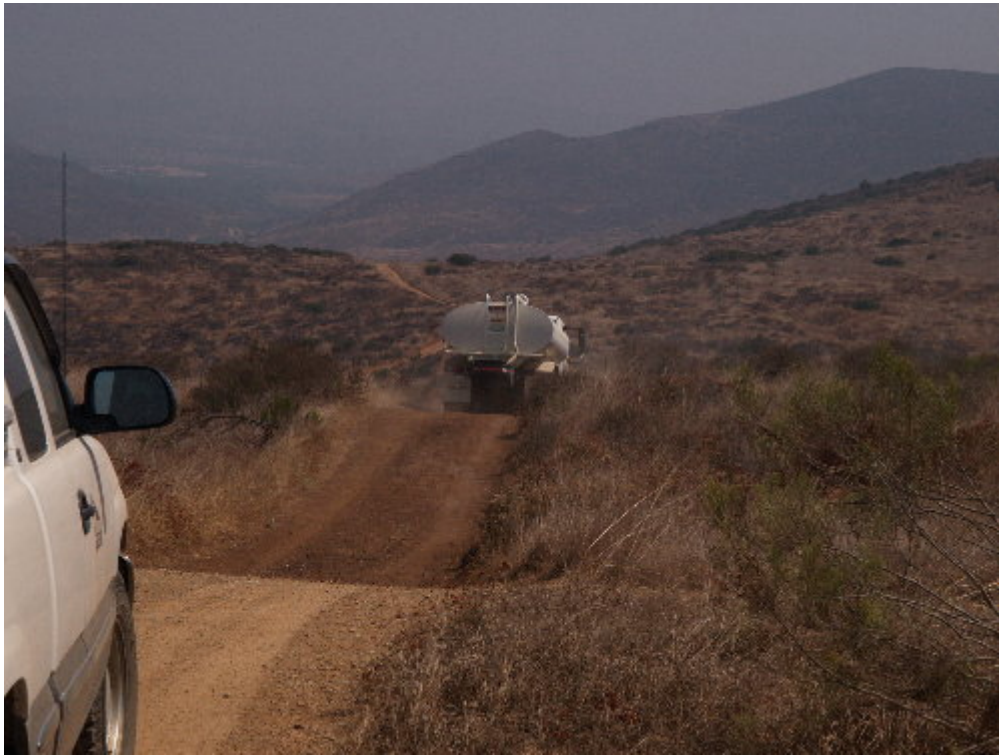
Figure 5 – A water truck worked to control dust in the Sweetwater area.
