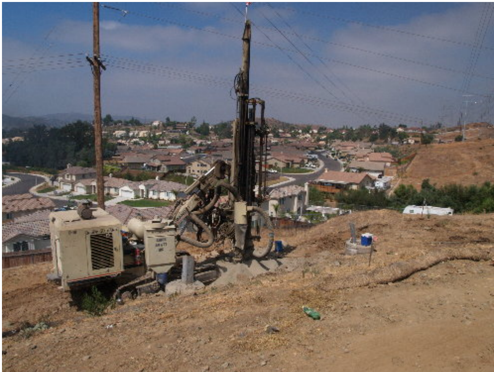
Figure 2 – Edick and Watt worked north of I-8 to test for rock with a small-diameter drill head.
