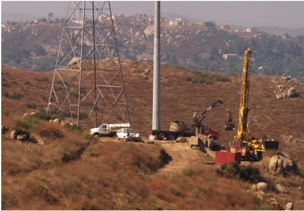
Figure 5 – The Tri-State Drilling crew worked on drilling at Tower Site 24.
