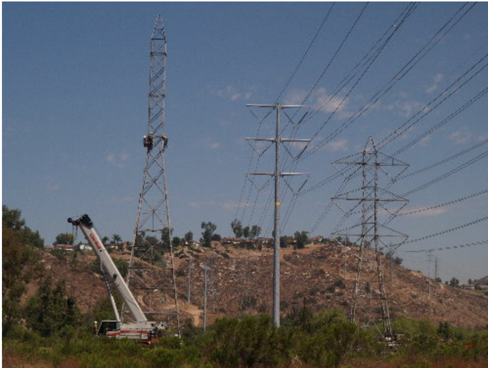
Figure 4 – The Wilson tower modification crew worked to prepare the lattice tower near the Herrick Center for modification.
