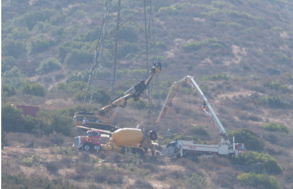
Figure 1 – The Tri-State drilling crew placed concrete in the excavation for Pole 58.
