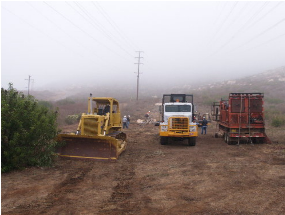
Figure 2 – The sagging operation was able to proceed despite the dense fog that moved in during the late afternoon.
