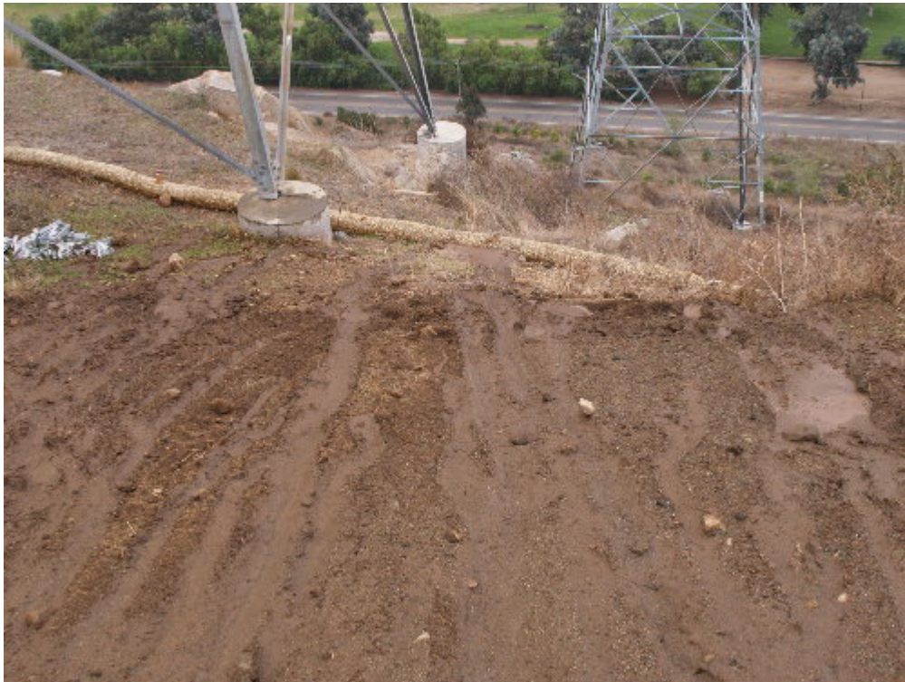
Figure 4 – The temporary BMPs at Tower Site 39 prevented erosion during the restoration process from entering the native habitat.
