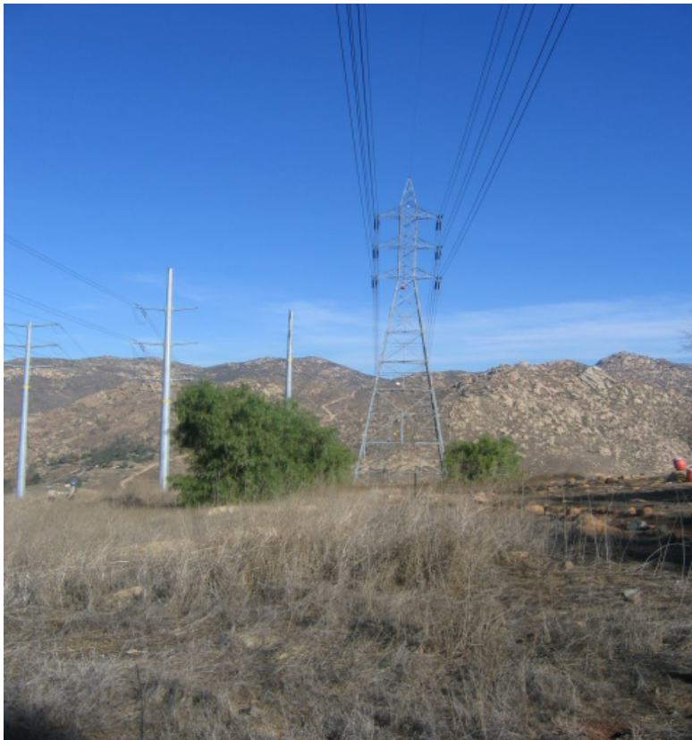
Figure 2 – Expanded stringing site located between Towers 576668 and 576669 to conduct stringing operations.
