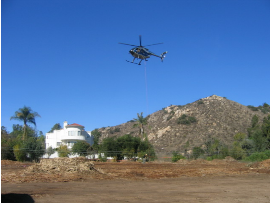
Figure 1 – Stringing operations between Towers 26 and 36 at Hillsdale Road.
