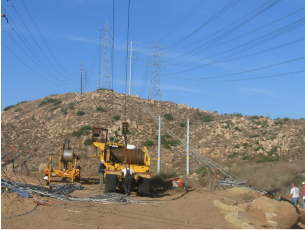
Figure 1 – Stringing operations continued between Towers 26 and 36.
