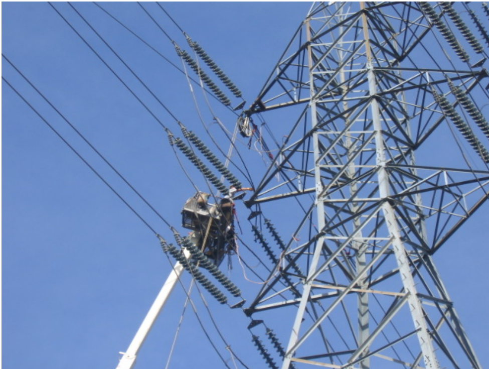
Figure 2 – Crews working to replace conductor over the San Diego River span.
