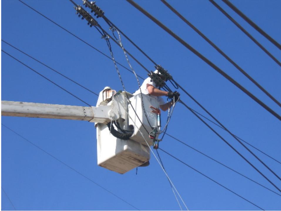
Figure 1 – Wilson worked on installing insulators above the Miguel Substation.
