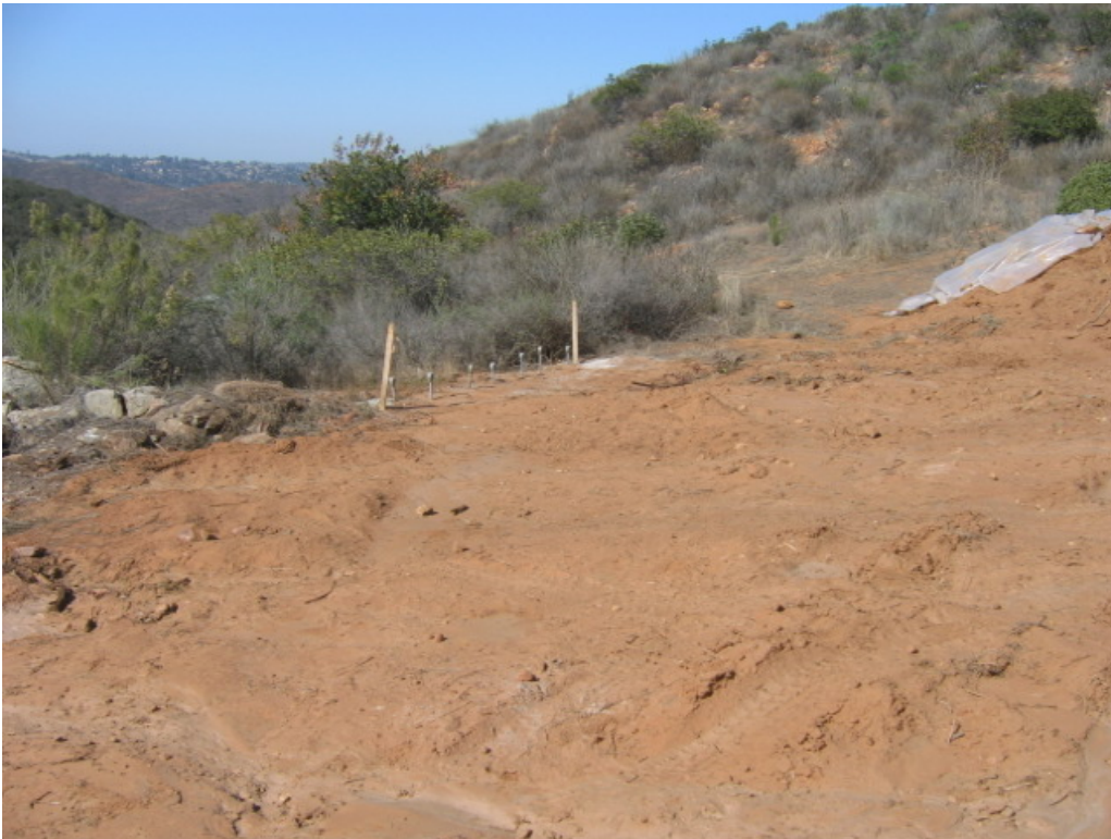
Figure 2 – Wilson crews will expand this existing stringing site near Site 52.
