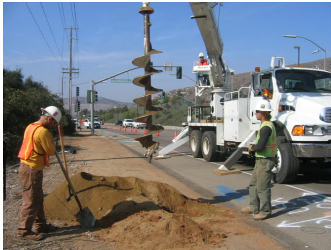
Figure 2 – Wilson crews installing guard structure to protect Highway 94.
