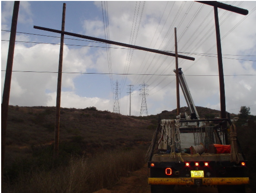
Figure 2 – Guard structure removal near Steel Canyon High School.
