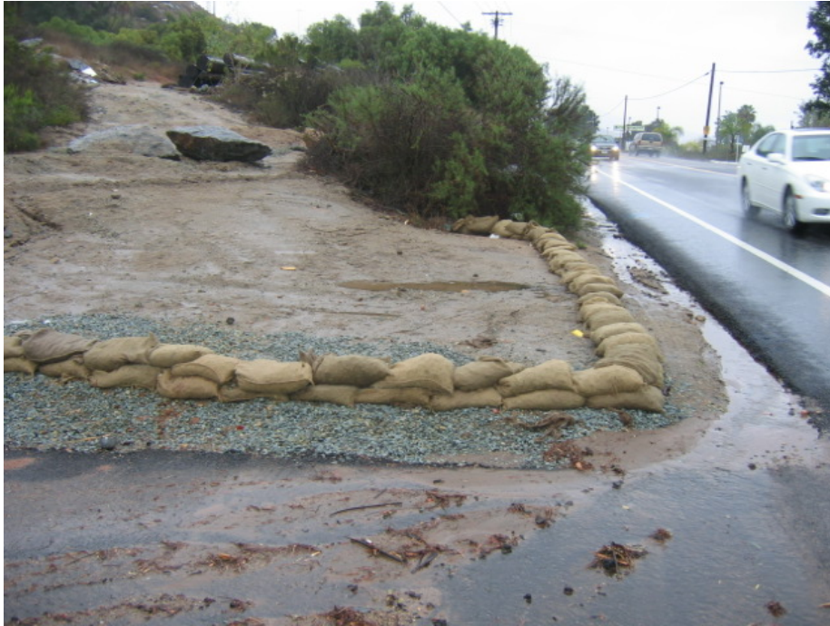
Figure 1 – BMPs in place along Willow Glen Road during rain event February 28 th .
