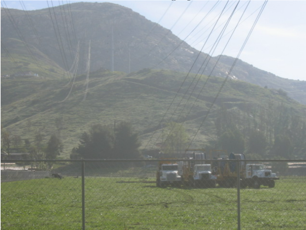
Figure 1 – PAR crews were set up near Willow Road in Lakeside to prepare for flying in the last section of rope.
