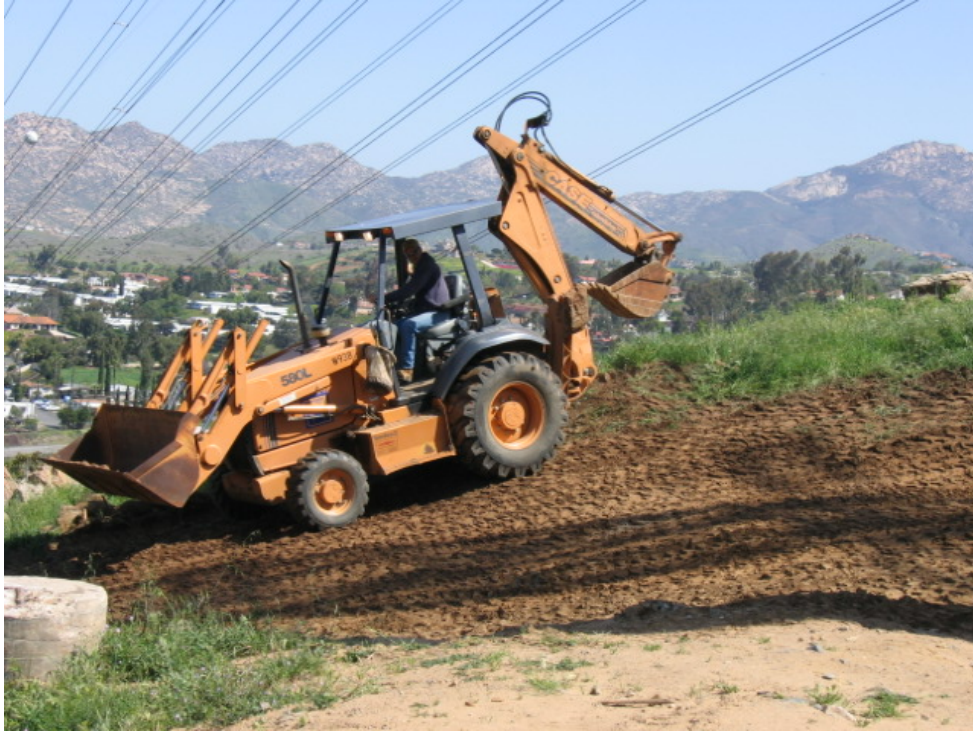
Figure 1 – Wilson crews recompacting a tower pad area near Highway 8.
