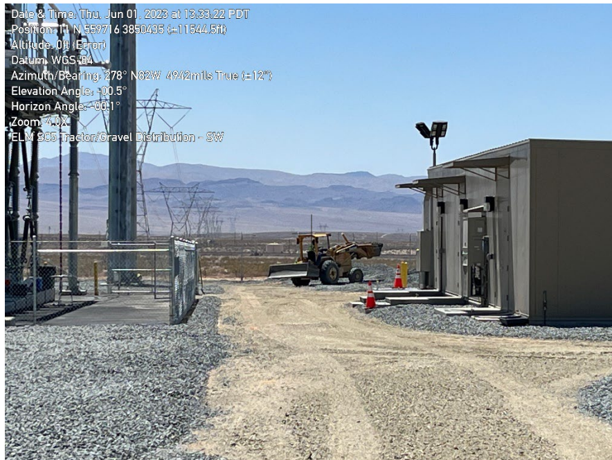
Photo 1: Backhoe activity (gravel distribution) at SC5, bringing site to final grade on June 1st.
